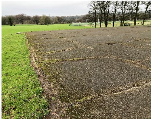
EXISTING – Old Macadam Surface
