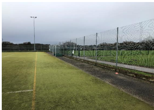
EXISTING – Sand Filled Synthetic Turf
