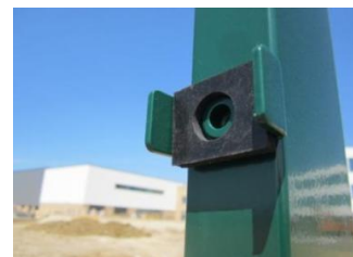
Neoprene washer within U shape fixing bracket
