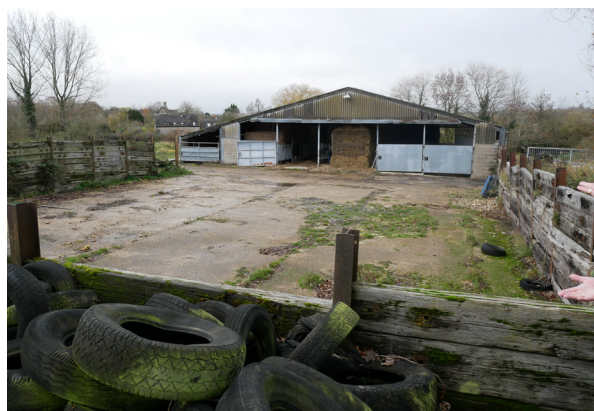
Fig 11. Eastern end of the Cow Shed and hard-standing.
