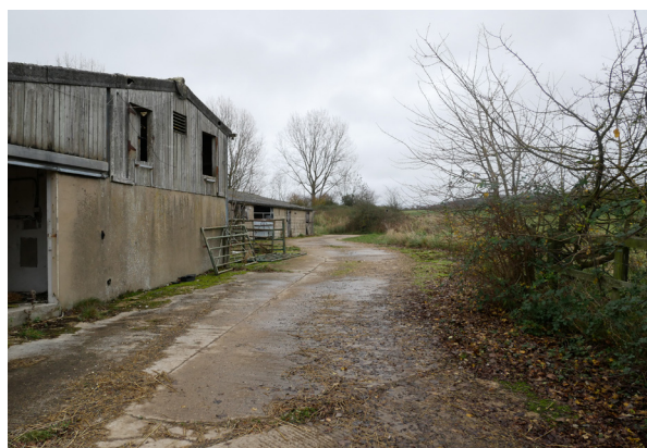
Fig 9. Southern aspect of the Cow Shed.
