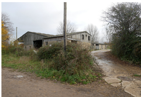
Fig 8. View into the site from Mill Lane.
