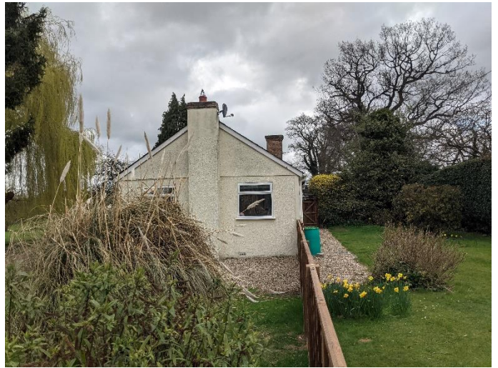
Photo 2 West elevation of bungalow
