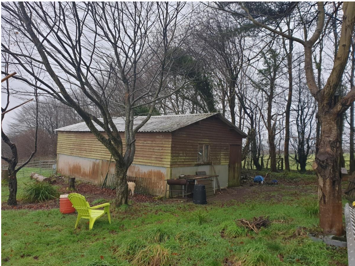
Northwest gable and northeast face.
