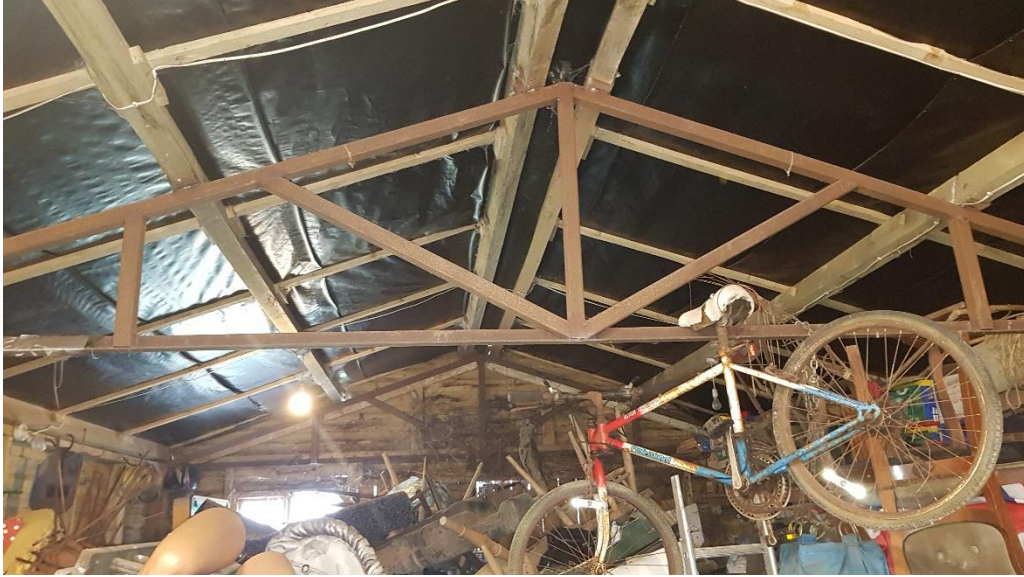
Photograph 1. Steel trusses to roof structure
