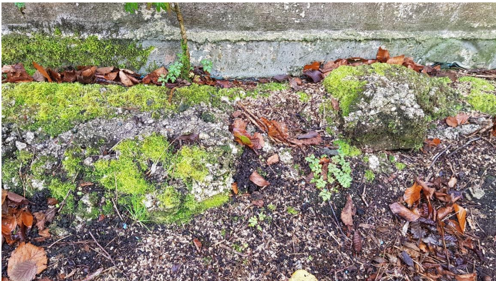
Photograph 2. Concrete slab and edge thickening
