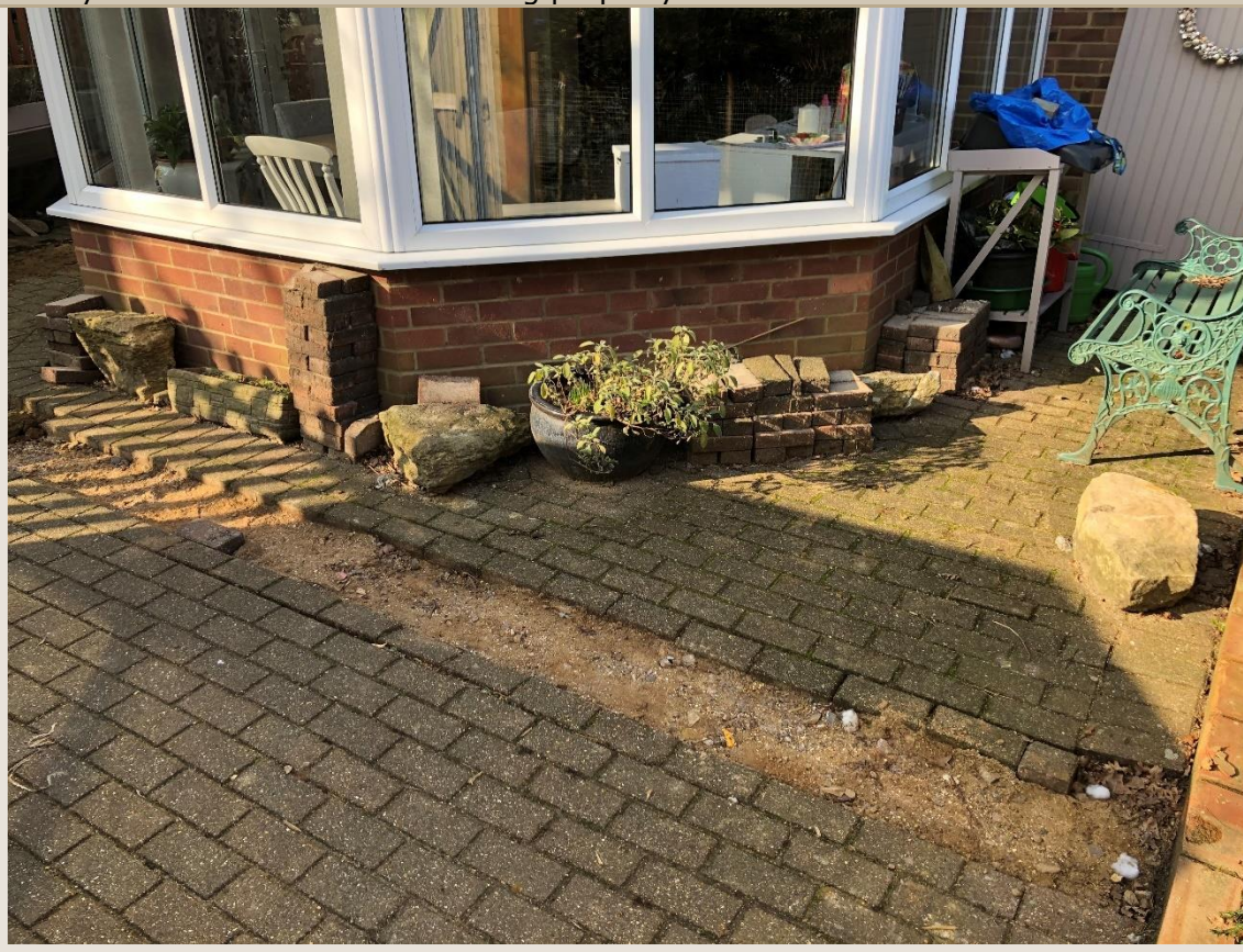
Air spade works in proximity to existing.
