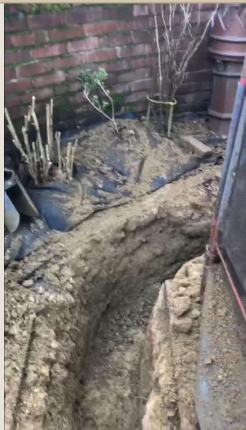
Air spade excavations on the corner closest to T1
