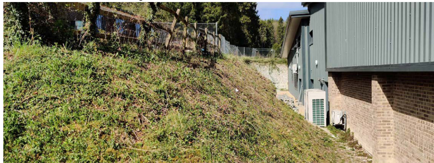
Photograph A - Site area - Westerly view from the maintenance access steps.
