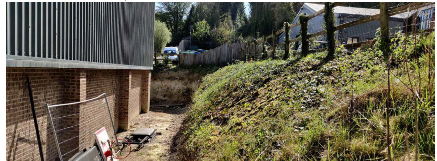
Photograph A - Site Area - Easterly view from the maintenance access steps.
