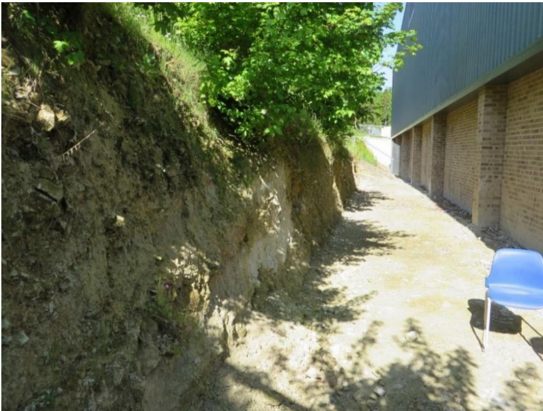
View 6: Rear of Sports Hall looking East.
