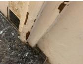
Fungal decay is always associated with a high moisture content in timber and therefore timbers bearing in or in contact with the walls where moisture has or may have penetrated must be considered suspect.
