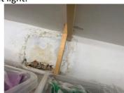
Further damp was notable behind the dry lined walls of the rear office after exposure works were carried out by others.
