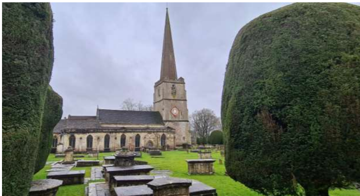
Plate 7: The Church of St Mary, Painswick Conservation Area
