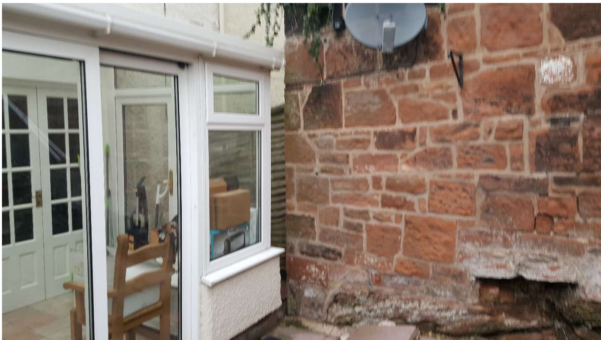
Image of the existing wall
