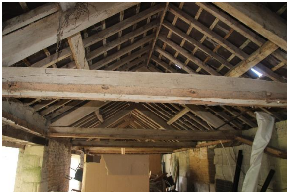
5. Interior of stock shed
