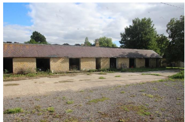
4. SW end of buildings from north
