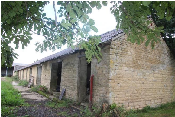
1. SW gable end of stock shed
