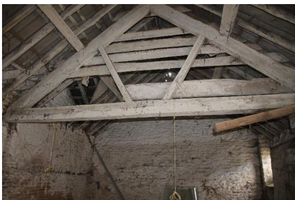
7. Queen post roof in NE building
