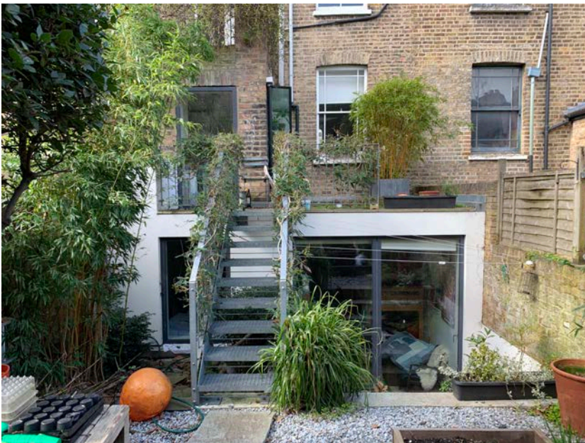
Rear of 12B Approach Road looking North-West.
