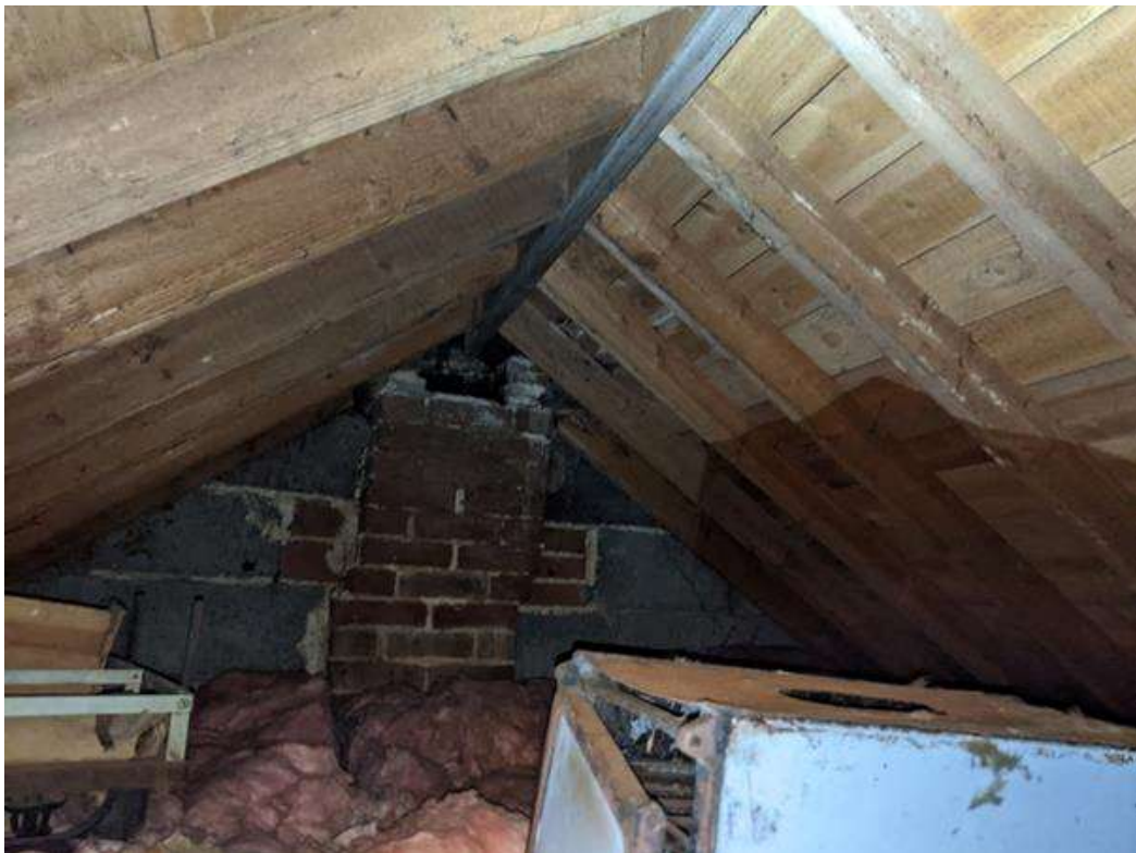
Photo 4 - View inside the main loft of the dwelling, with tight timber sarking.
