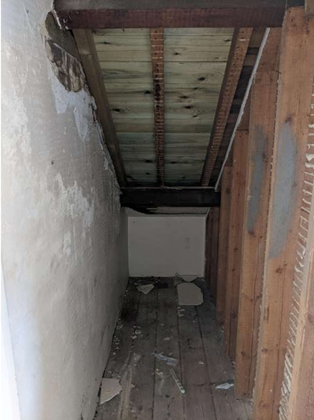
Photo 5 - The walk-in roof space to the north of the dwelling.
