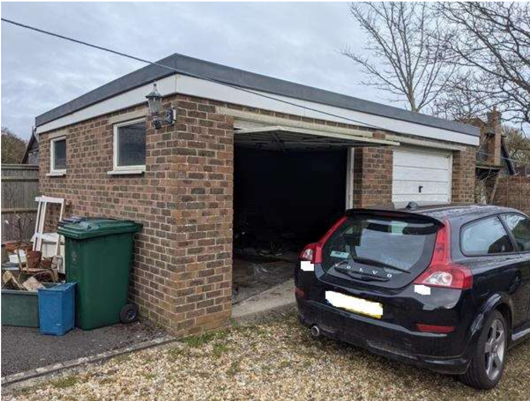
Photo 3 - View of the garage building.
