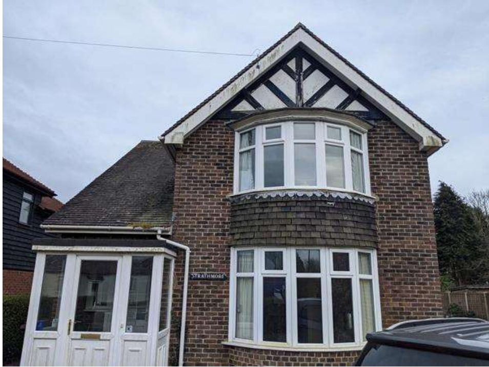
Photo 1 - View of the dwelling from the west. The dormer window is proposed to be pitched roof to the left, whilst hanging tiles to the main building would be replaced.
