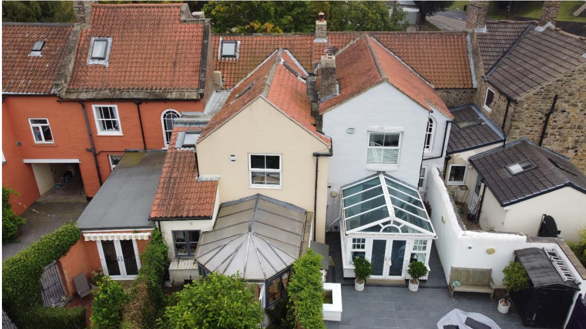
Figure 3 – Rear of 30 High Bondgate (No. 28 to the left)
