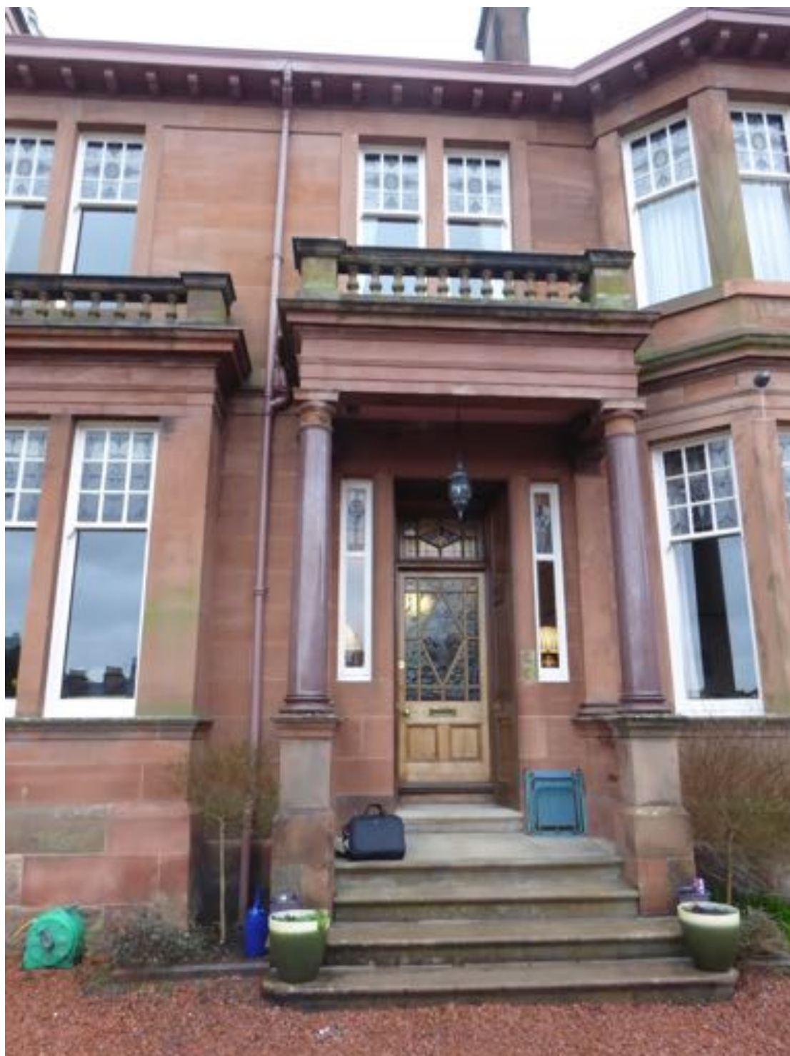
3. View of Entrance Portico with New Downpipe to South of Entrance
