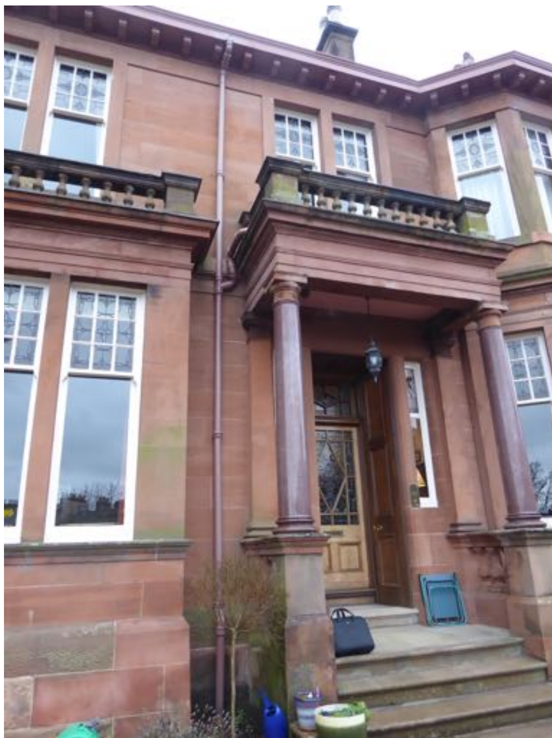
4. View of New Downpipe to South of Entrance
