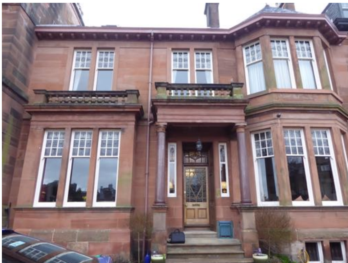
2. View of East Elevation from East
