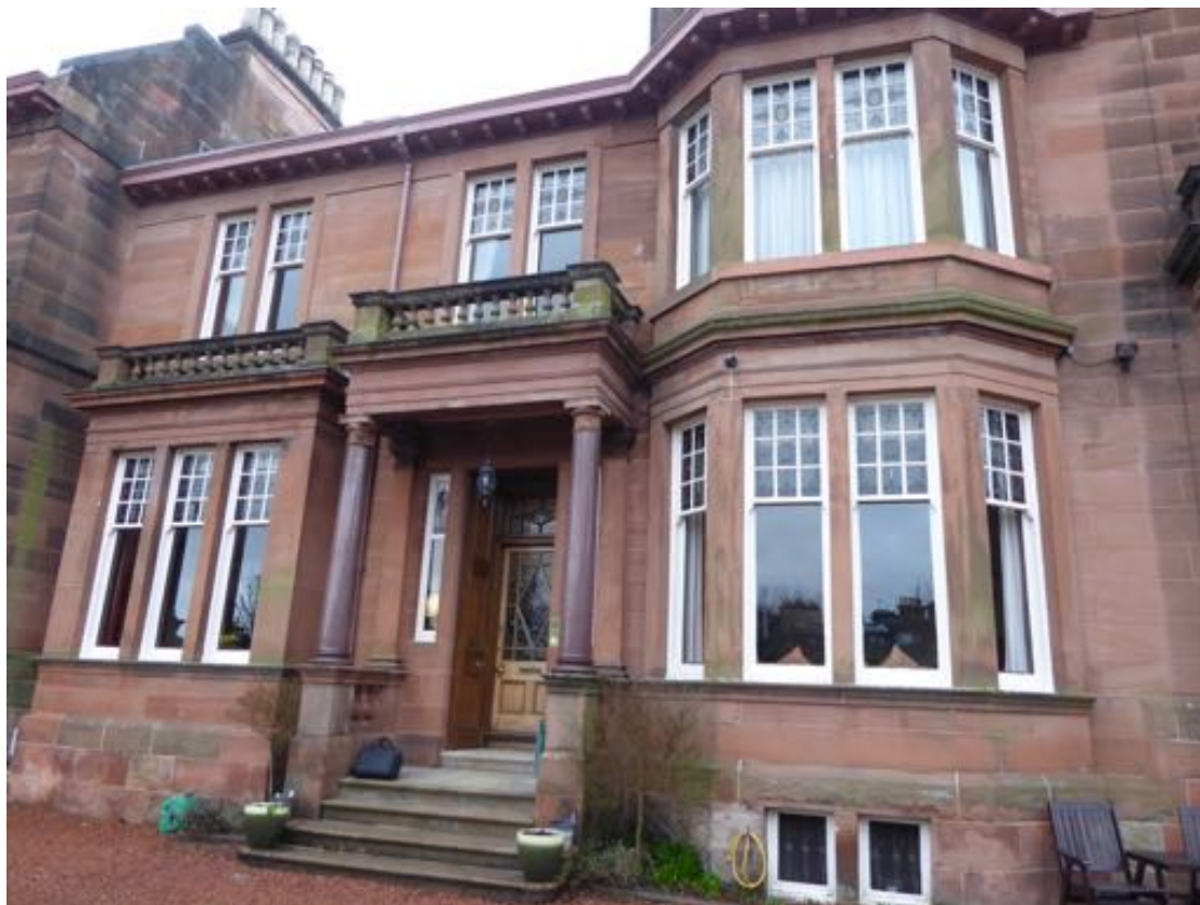
1. View of East Elevation from Northeast
