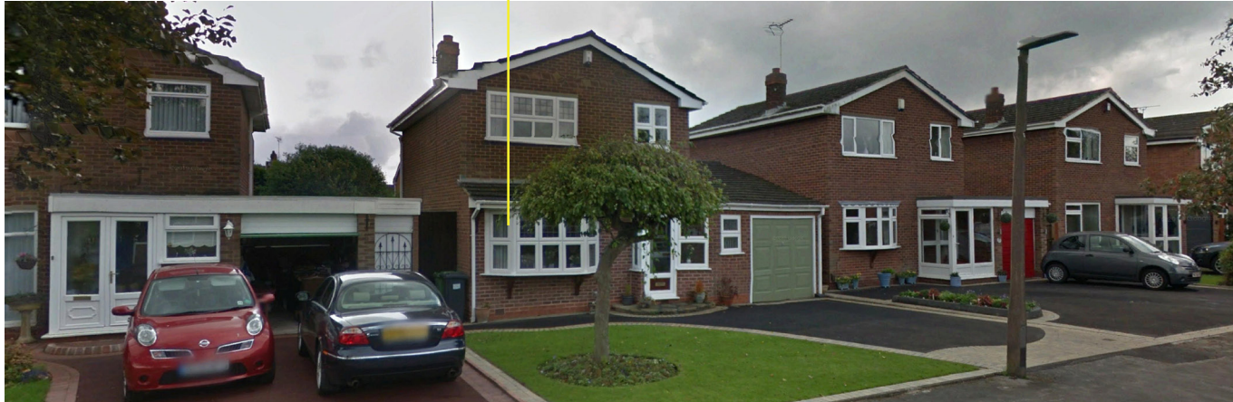
Northern Street Elevation down Hansell
