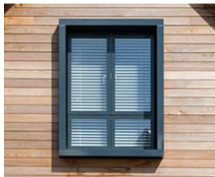
Example of aluminium windows
