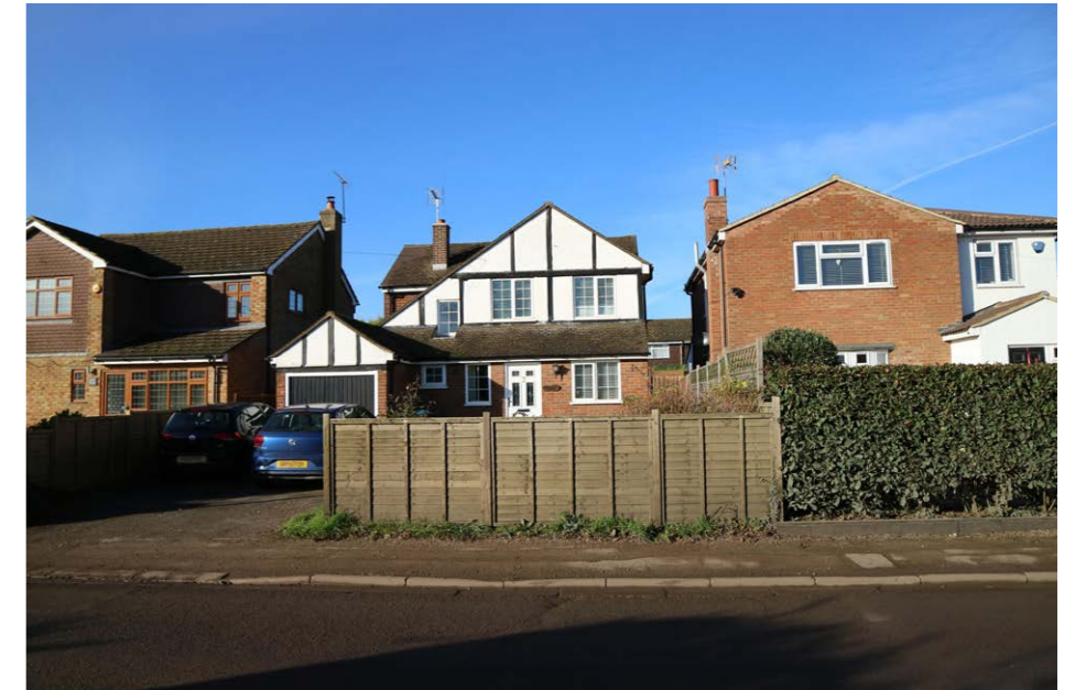
Detached Houses - 20-22 Chesham Road Materials - Brick, Render and Timber detailing, Brown Timber Weatherboarding, White and Brown Fenestration.
