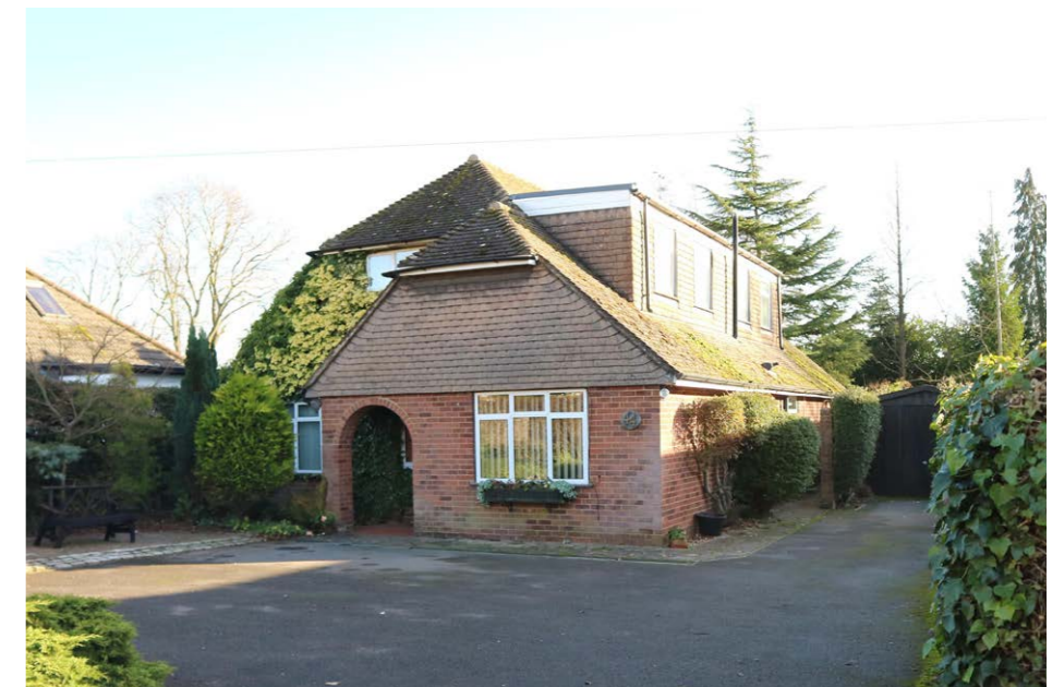
Detached Bungalow - 44 Chesham Road Materials - Brick and Timber Weatherboarding with White Fenestration
