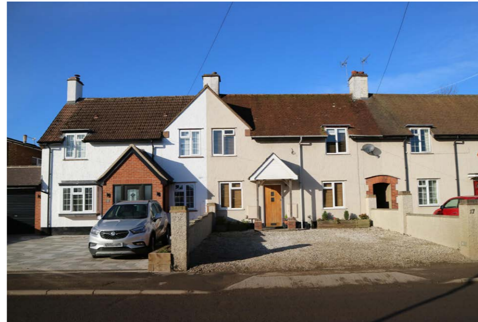
Terraced Houses - 16-18 Chesham Road Materials - Different Coloured Render, White Fenestration with Clay Roof Tiles of Different Shades.
