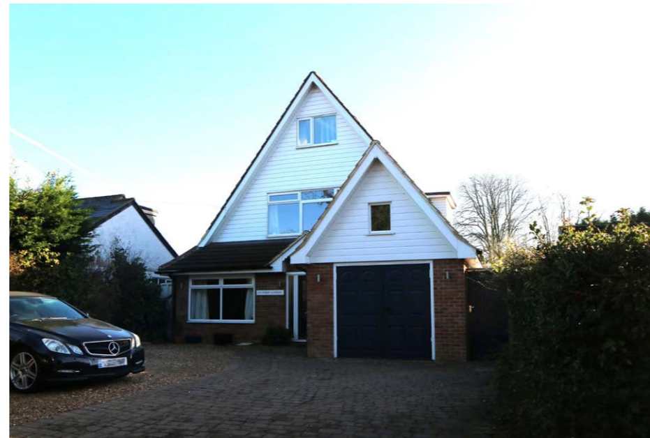
Detached Chalet Bungalow - 40 Chesham Road Materials - Brick and White Timber Weatherboarding and Fenestration
