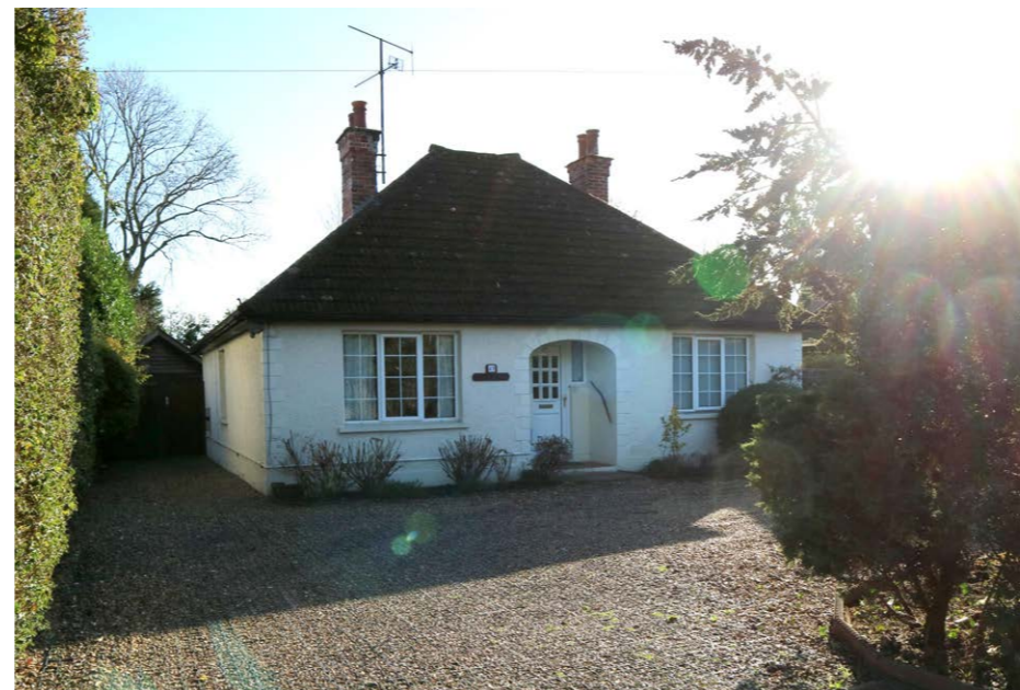
Detached Bungalow - 47 Chesham Road Materials - Render with White Fenestration and Dark Clay Roof Tile
