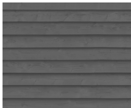
Example of stained timber boarding
