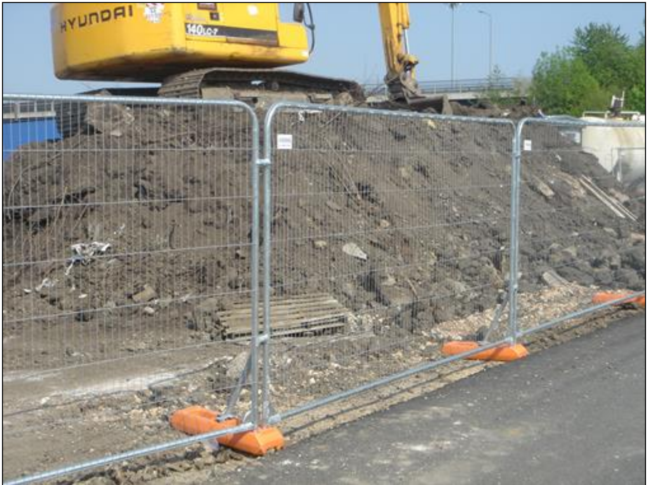
Photograph C – Example of Heras Tree Protective Fencing
