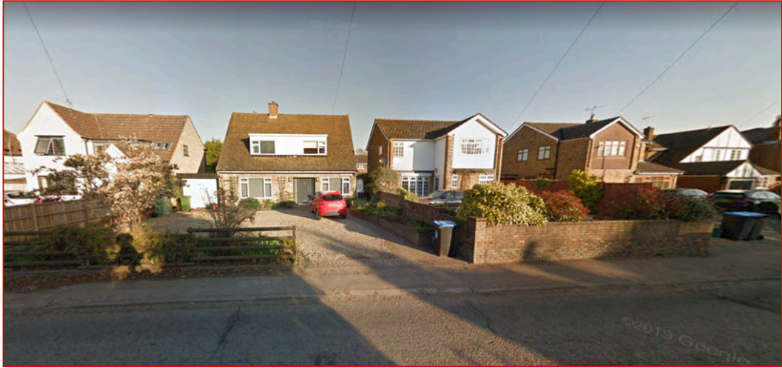
Figure 7.0: Detached dwellings on the western side of Chesham Road
