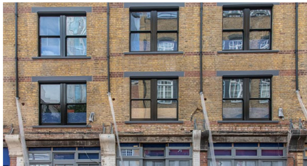
Dark grey lintels and ledges opposite the site at 10 Cobb Street (Chris Dyson Architects)
