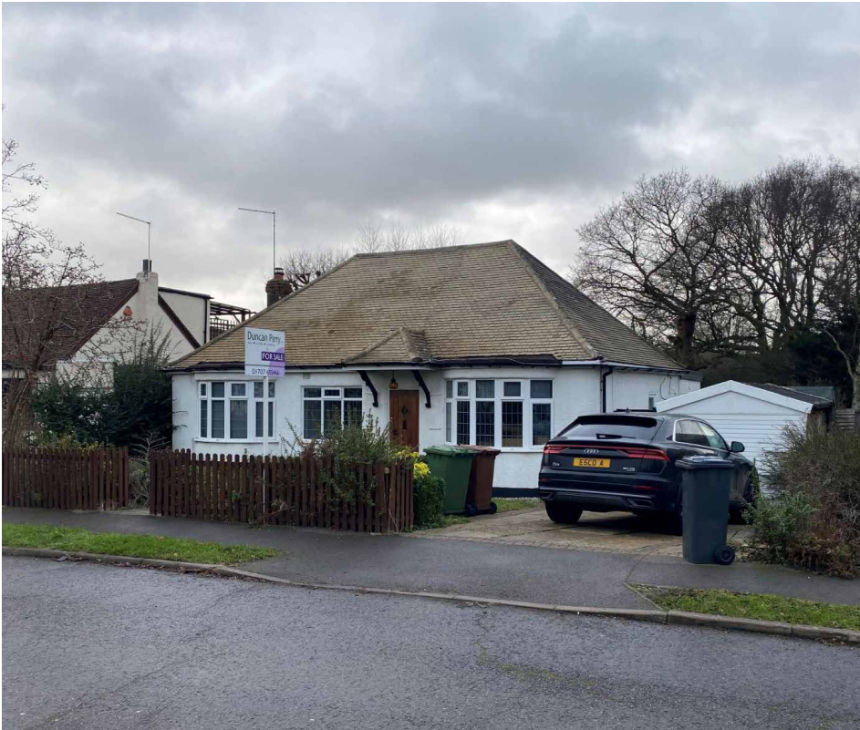
Existing street view
