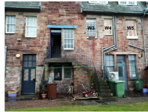
Rear Elevation Photo
