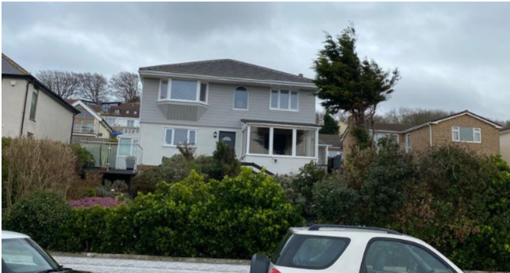
Above: Front of no 43 and previous split plot development 45 and 45a
