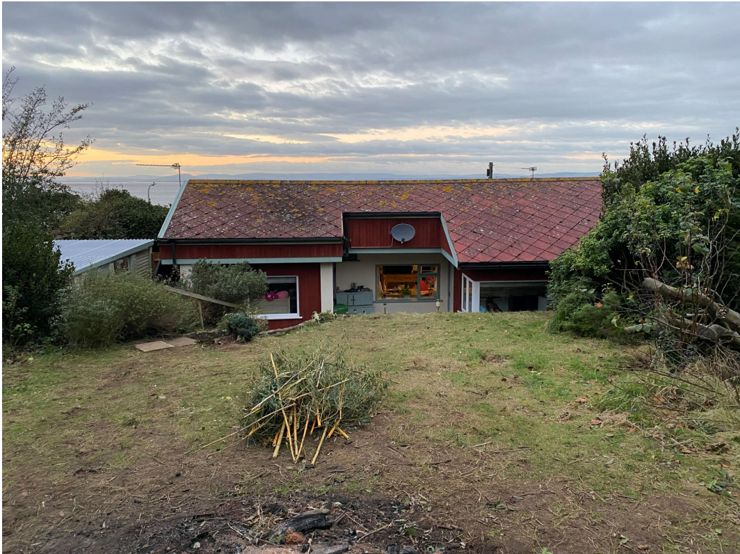
Above: Rear of existing property from garden level
