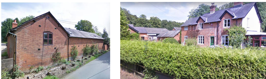
Figure 3 – Two photos of the site taken from Old Odiham Road
