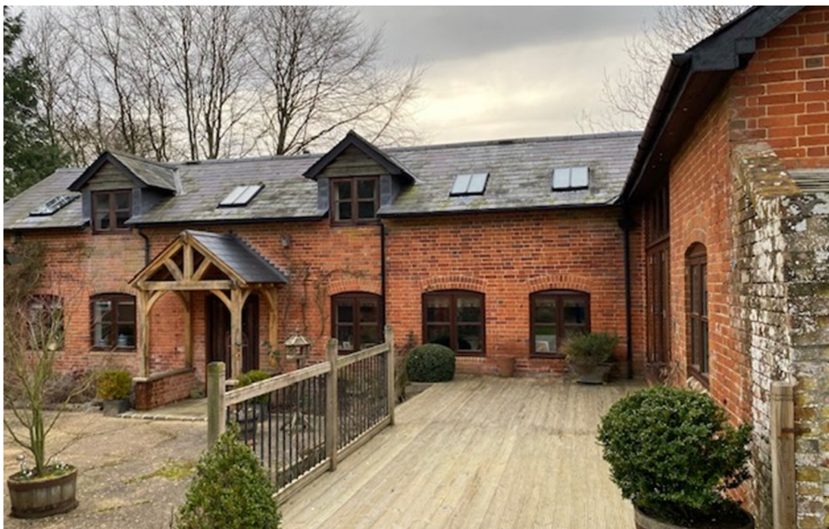
Figure 2 – Photograph taken 2021 of the Barn
