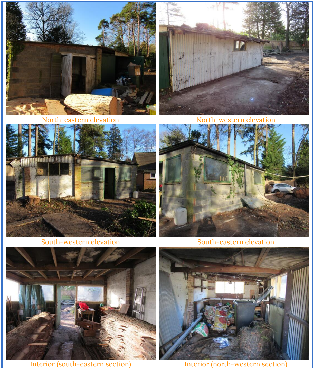
Figure 4-2: Photographs of the garage
