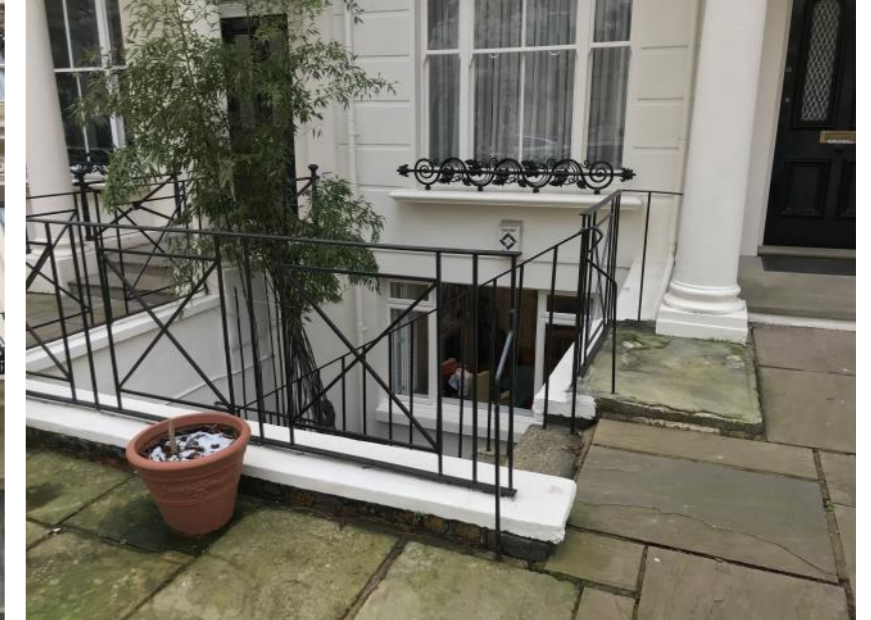
METAL RAILINGS TO LIGHTWELL
