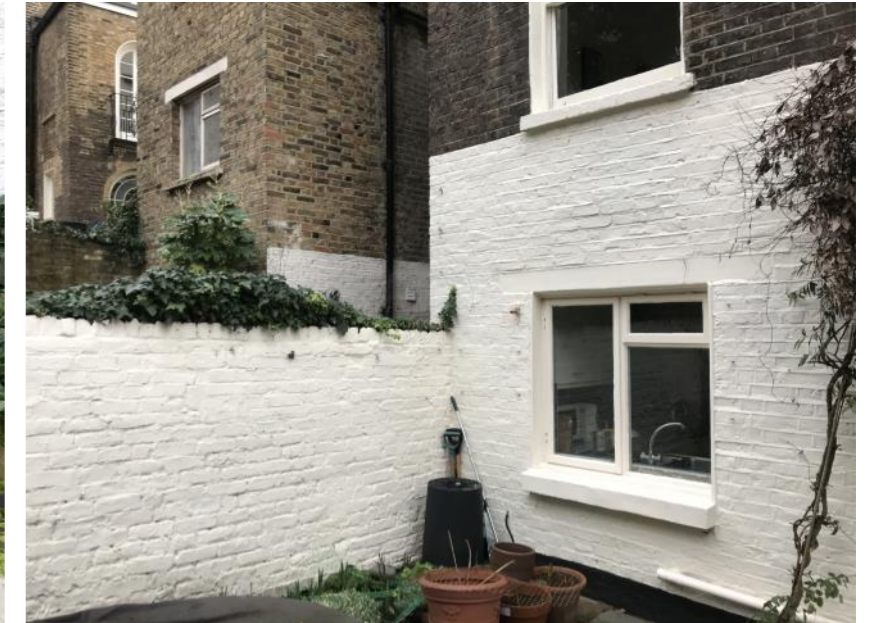
CLOSET WING, NON ORIGINAL LOWER GROUND FLOOR WINDOW
