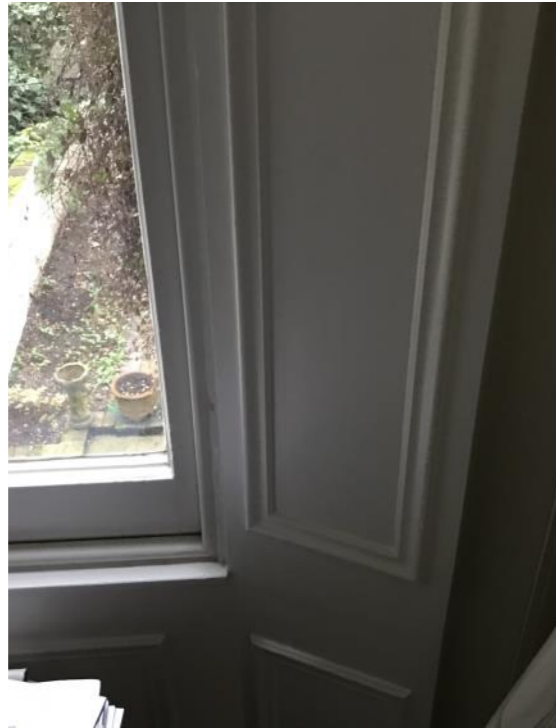
ORIGINAL SHUTTERS TO FRONT AND REAR BEDROOMS
