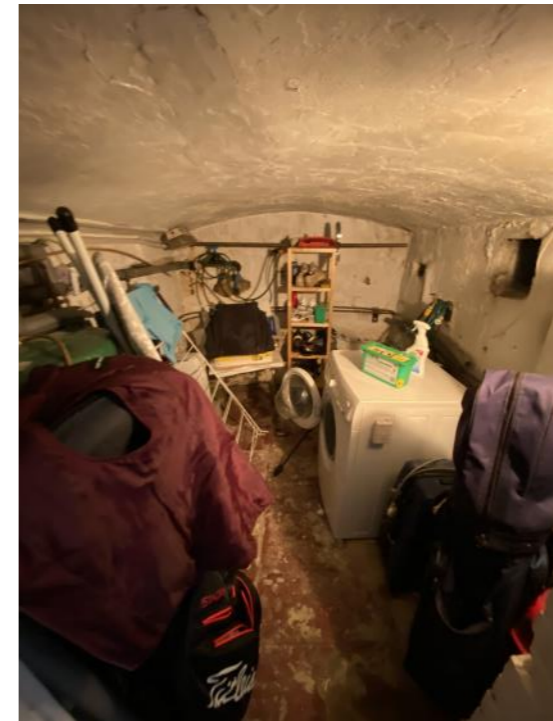
LOWER GROUND FLOOR VAULT
