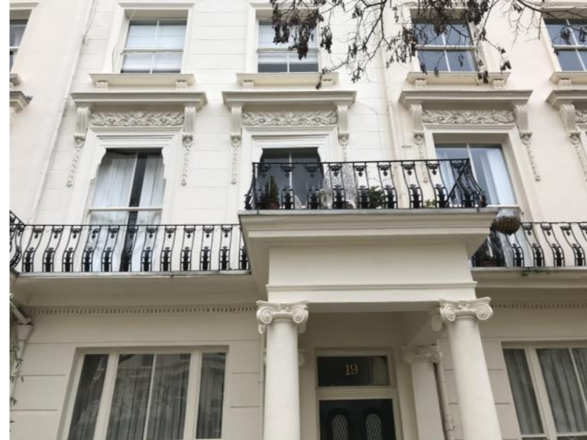
METAL RAILINGS TO FIRST FLOOR
