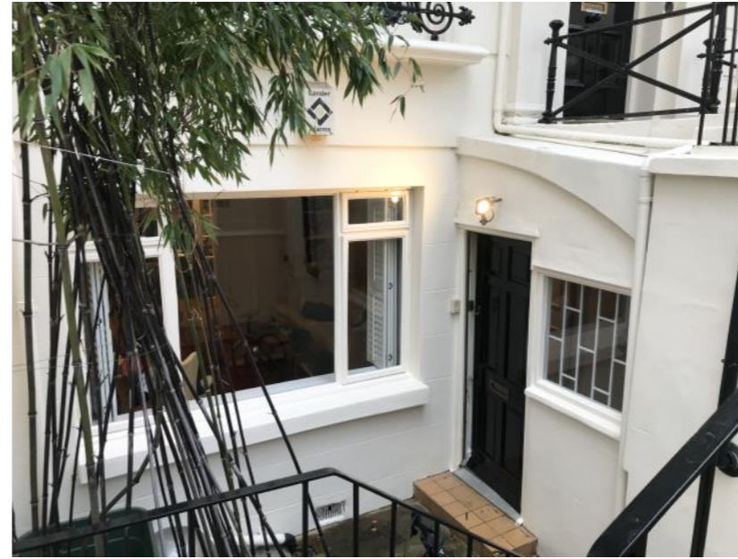
LOWER GROUND FLOOR LIGHTWELL
