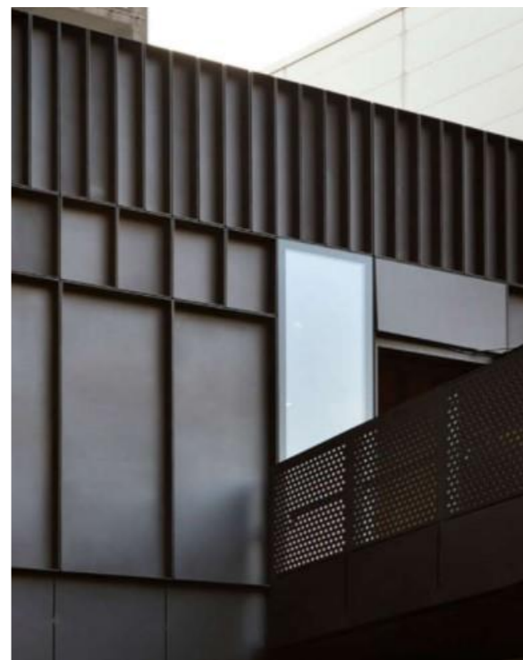
MORRIS+COMPANY—SHEPHERDS BUILDING— PROFILED METAL CLADDING
