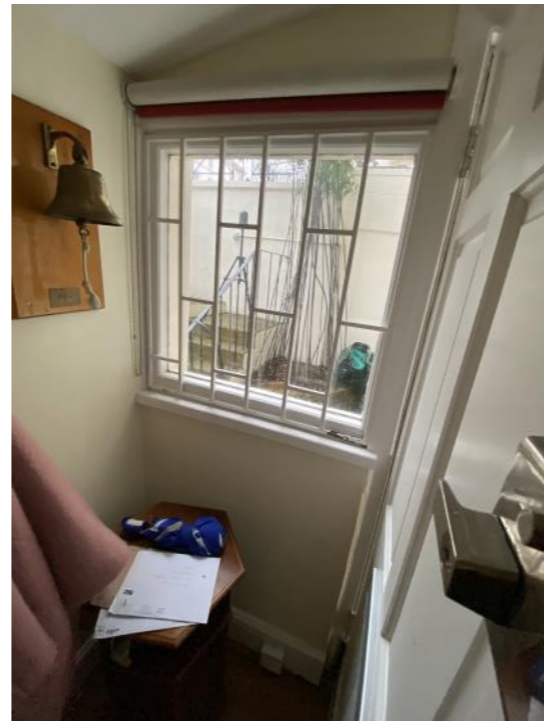
LOWER GROUND FLOOR PORCH
