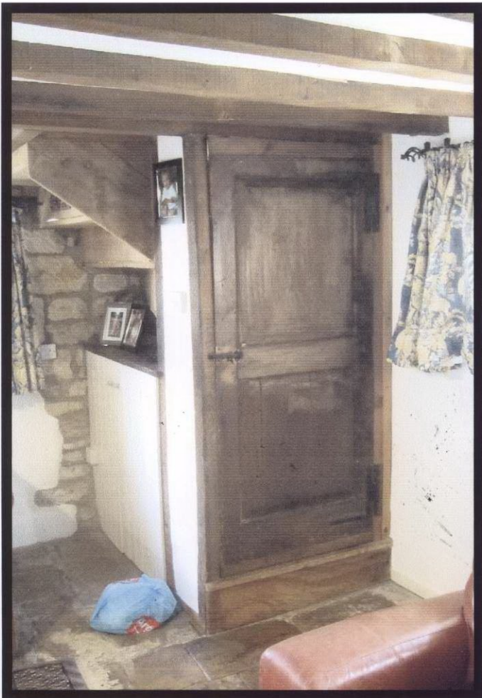
(2) Stairs to be removed showing door
