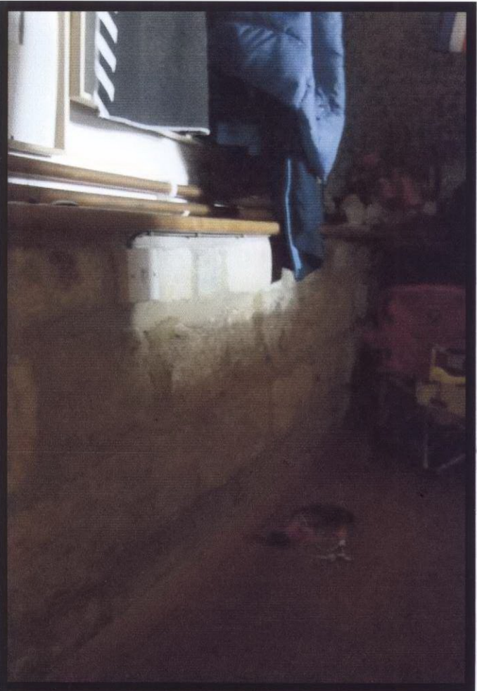
9 Dwarf wall from Bedr'm 1 (shwr Rmside)
