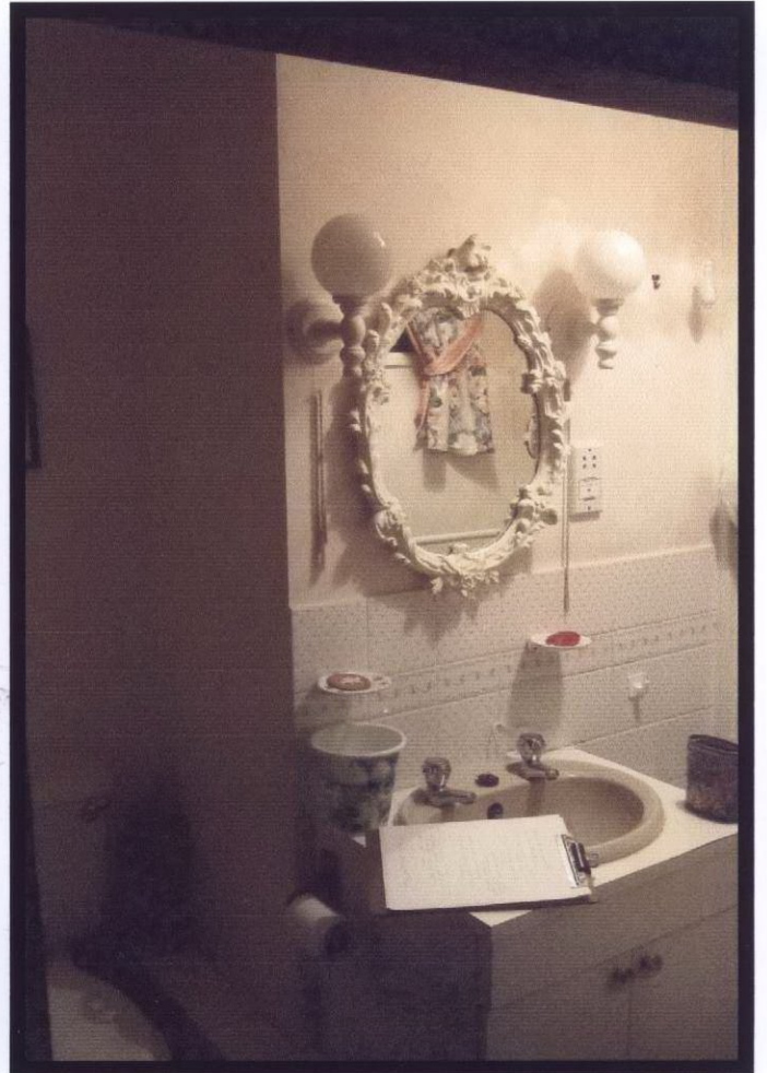
(13) Solid Bathroom Partition to be removed
