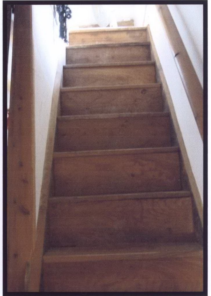
(12) Attic stairs (new) to be removed
