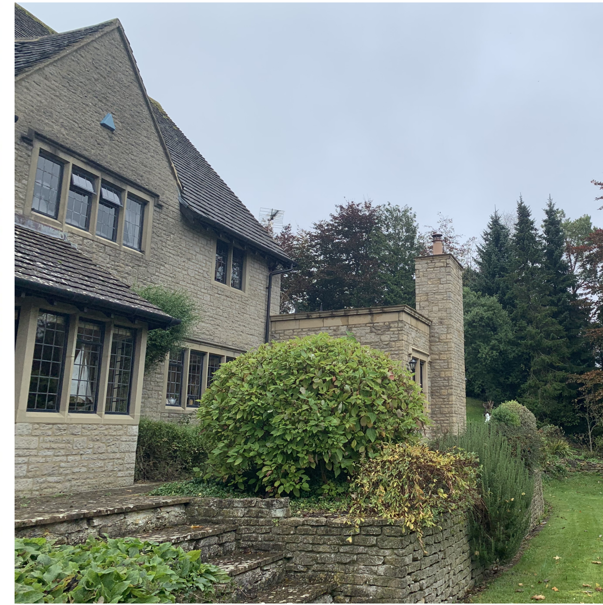
03 - STEEL FRAMED LEADED WINDOWS, BLACK FRAME & HARDWARE BY LOCAL FABRICATOR TO MATCH EXISTING PROFILE & PROPORTION OF WINDOWS TO EXISTING HOUSE, DOUBLE GLAZED. SITE MEASURED
