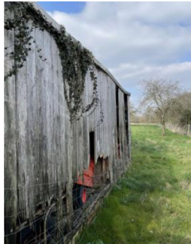
Rear of Stables East facing
