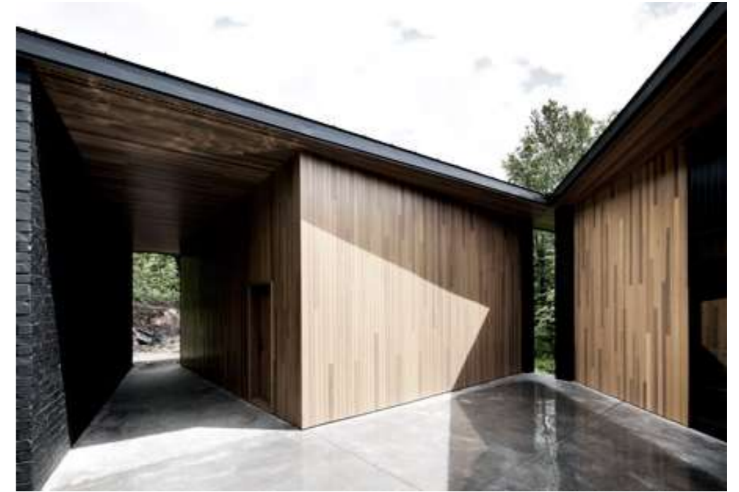
Timber cladding such as Western Red Cedar naturally weathers to a silver and provides a natural soft material palette.
