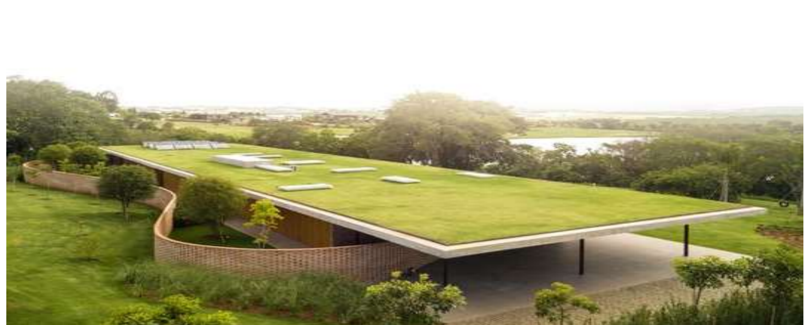
Reduced impact: Additional to the ecology benefits the green roof reduces the impact of the building merging into the landscape.
