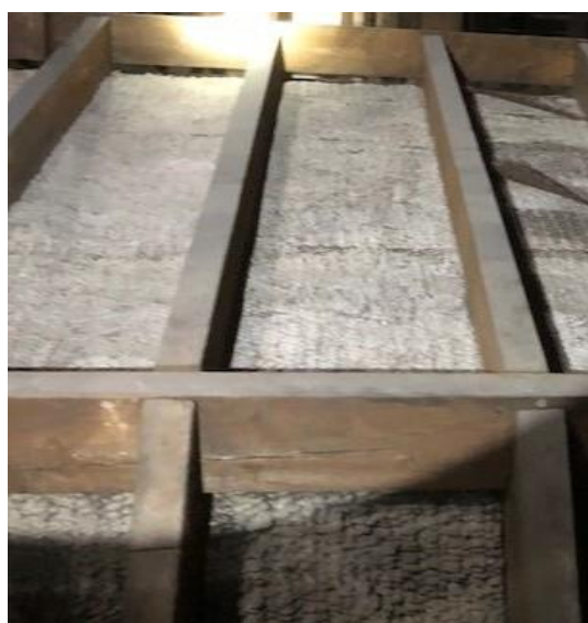
Rear of vaulted ceiling – Key in sound condition.
