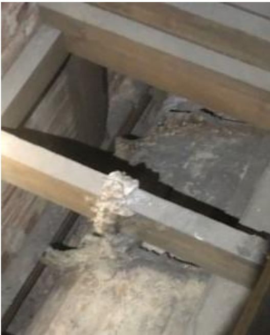
Wad to stage moulding – sound condition.
