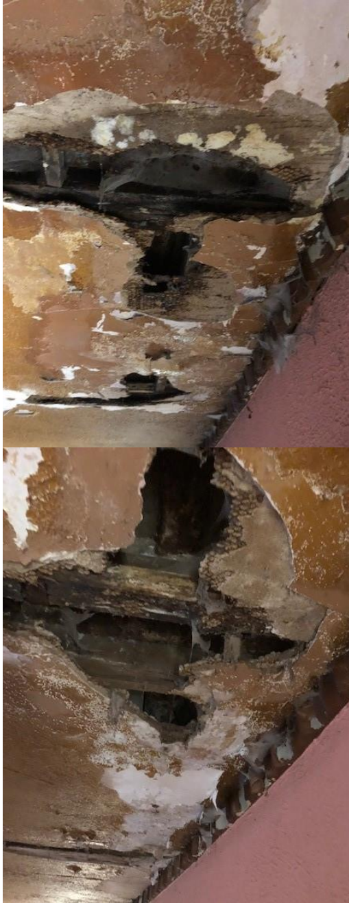
Ceiling to rear of stalls
