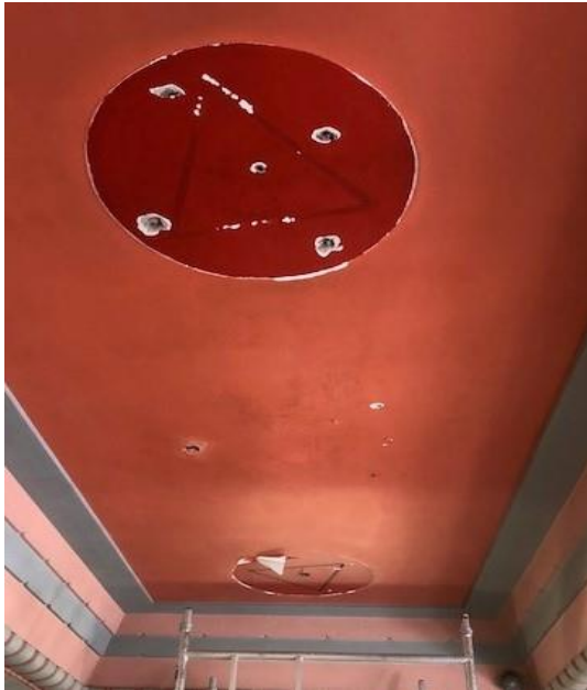
Main Lath & Plaster ceiling, view from Foyer.
