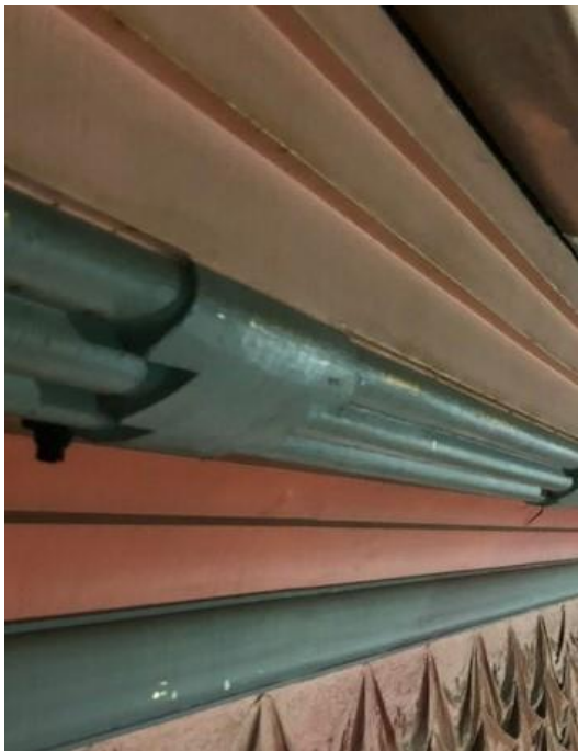
Front Pic. Good condition.
