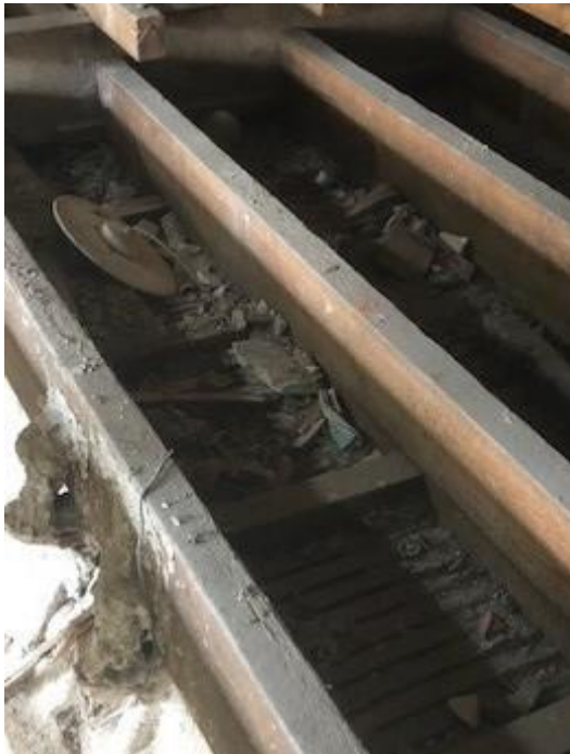
Main Lath & plaster ceiling – view from behind
