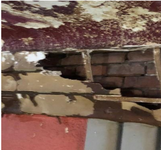
Cornice showing exposed timber lath
