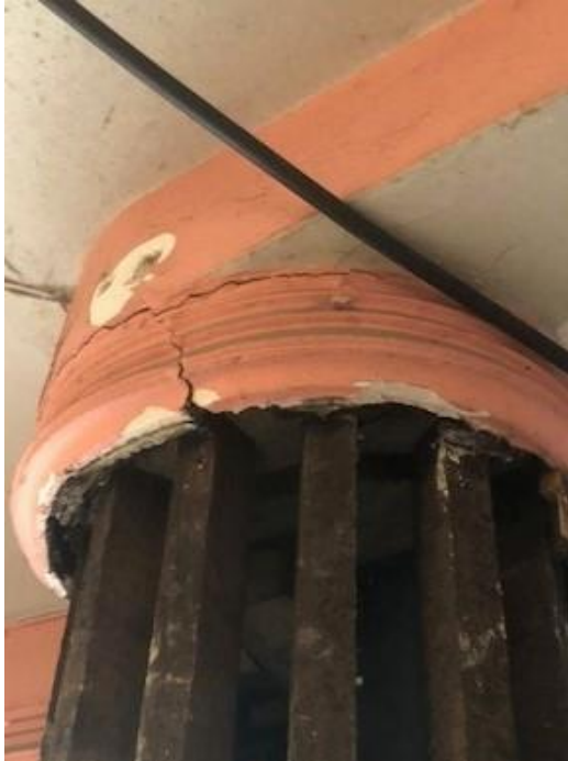
Curved / radius mouldings bottom of staircases in Foyer.
