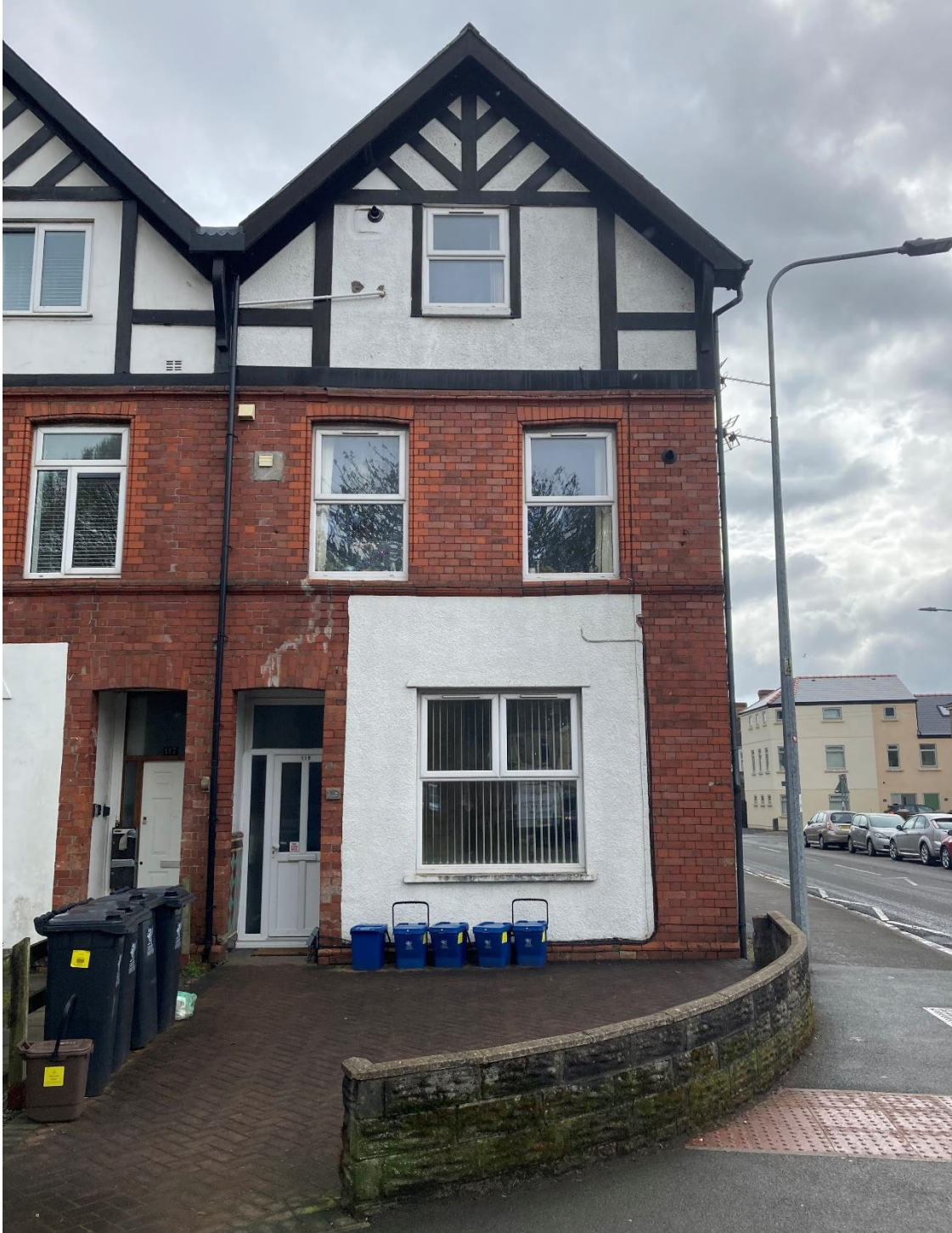
Figure 1: 119 Romilly Road north ('front') elevation
