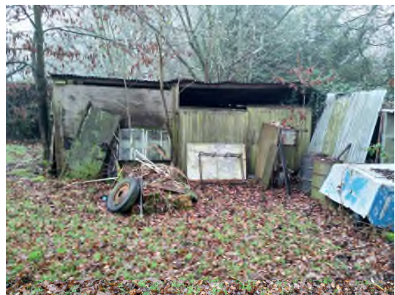
Image 2: The site contains various structures and sheds on site.
