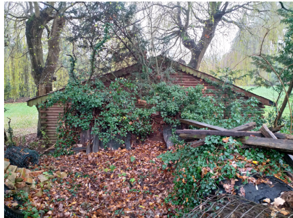
Image 6: The residential outbuilding at The Glen is clearly visible from the application site.
