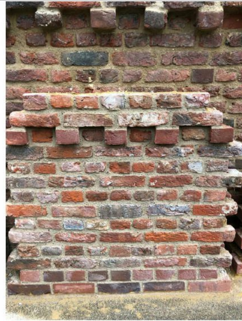
With Lime mortar pointing completed
