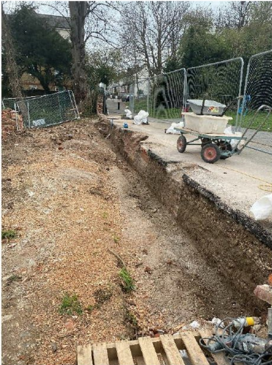
Looking East all bricks carefully removed
