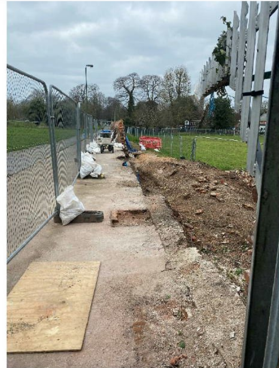
Looking West along the dismantled section
