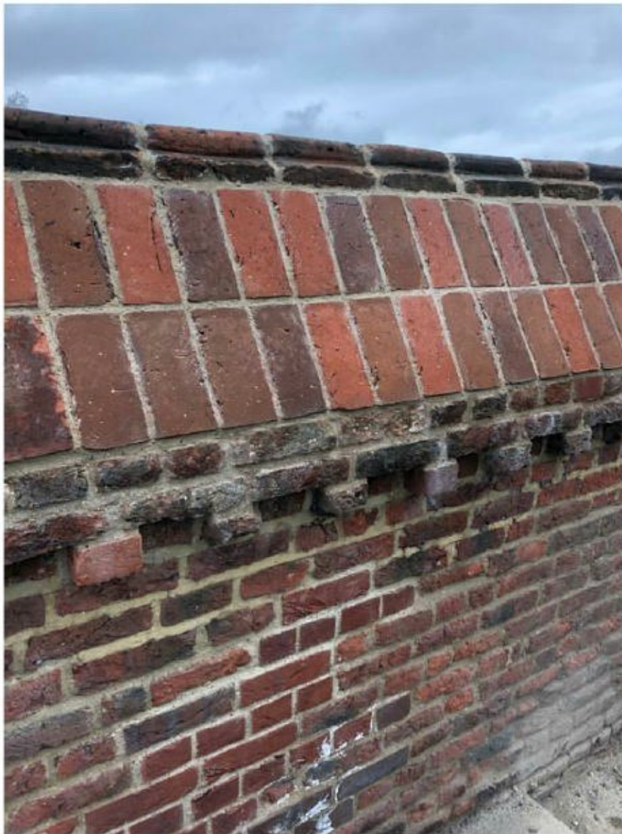
Shows the Goodwood brick to the skewed capping
