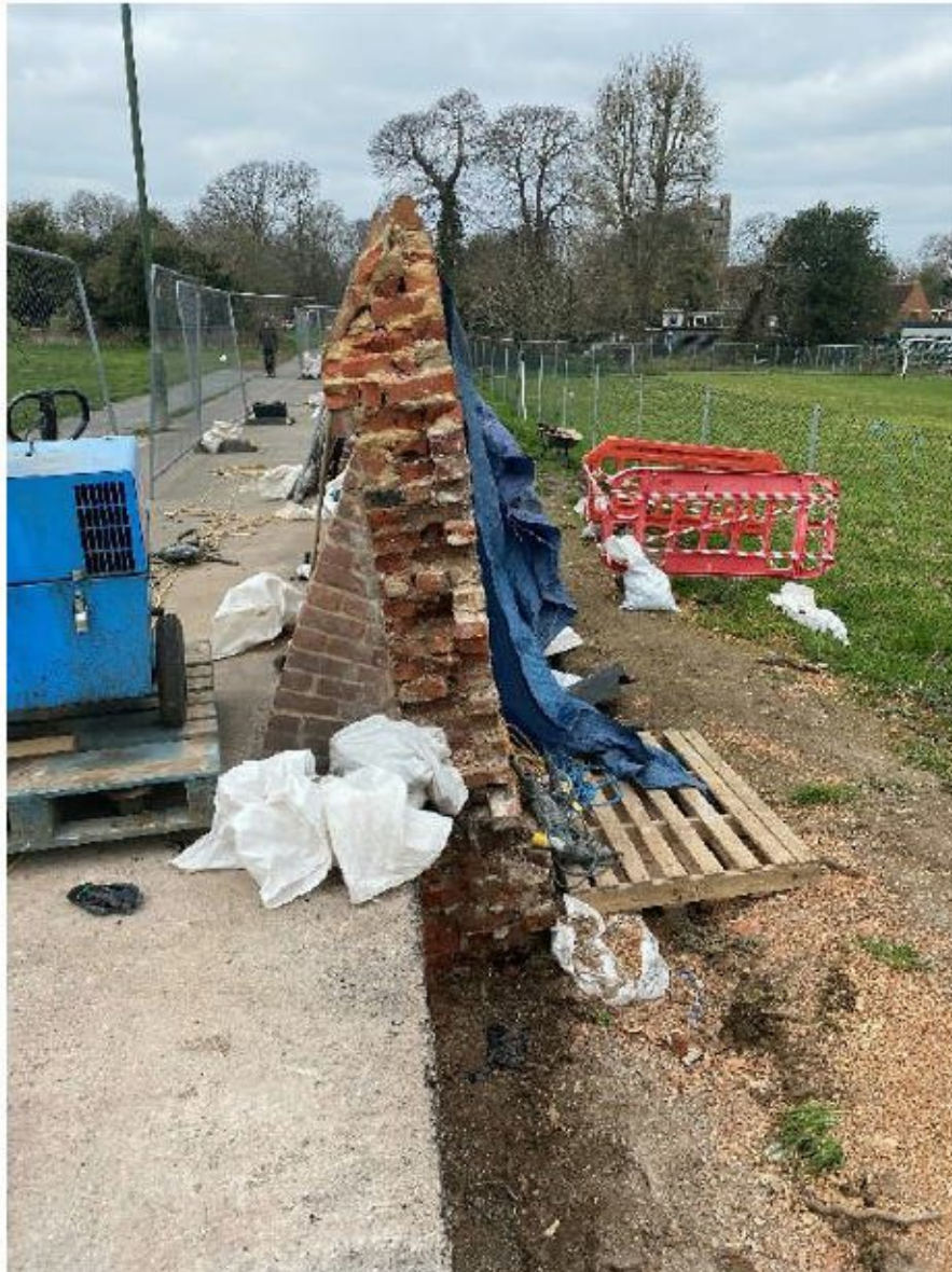
Dismantled to Buttress 8 Looking West
