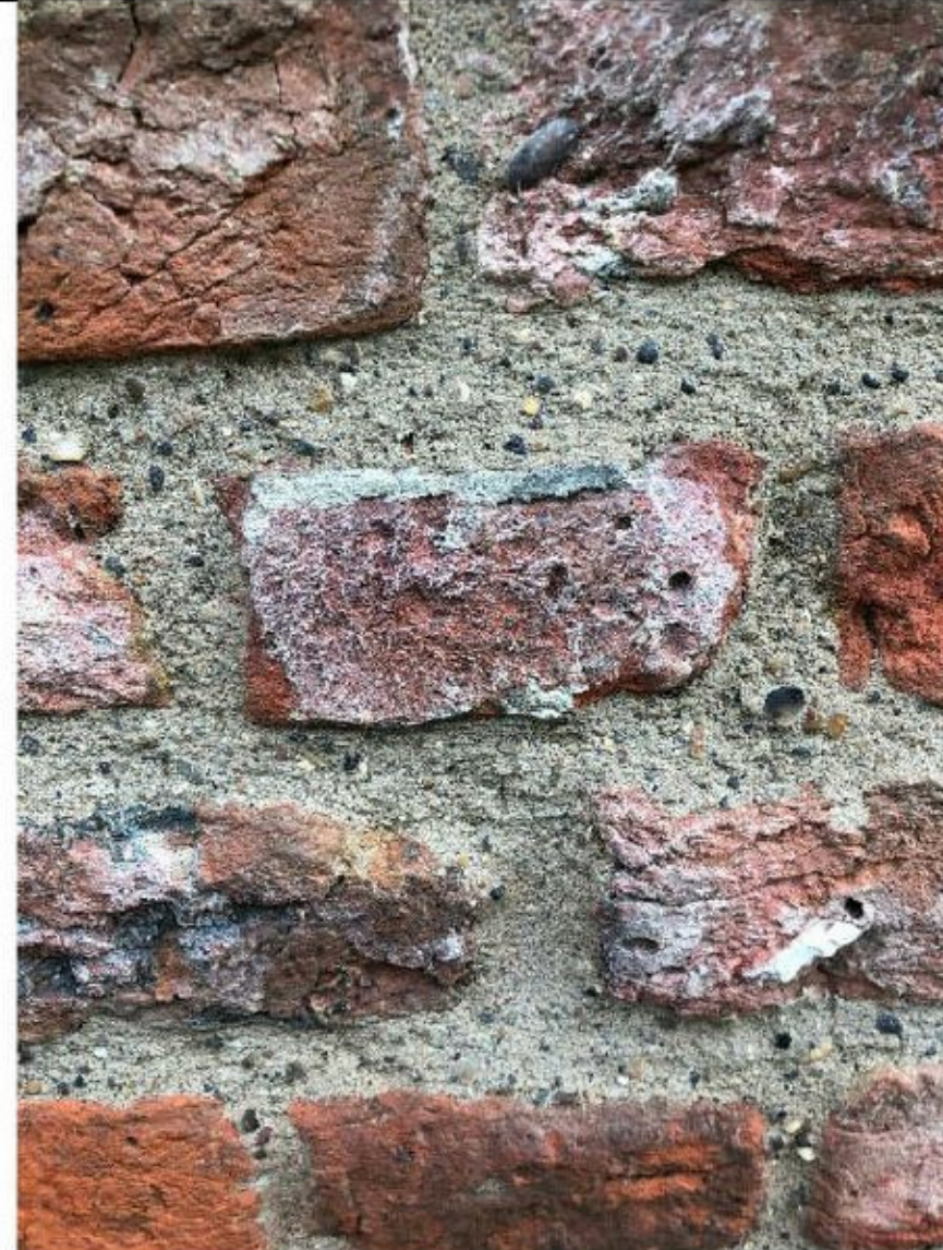
Shows Hydraulic Lime Mortar Proposed Pointing to Salvaged Bricks
