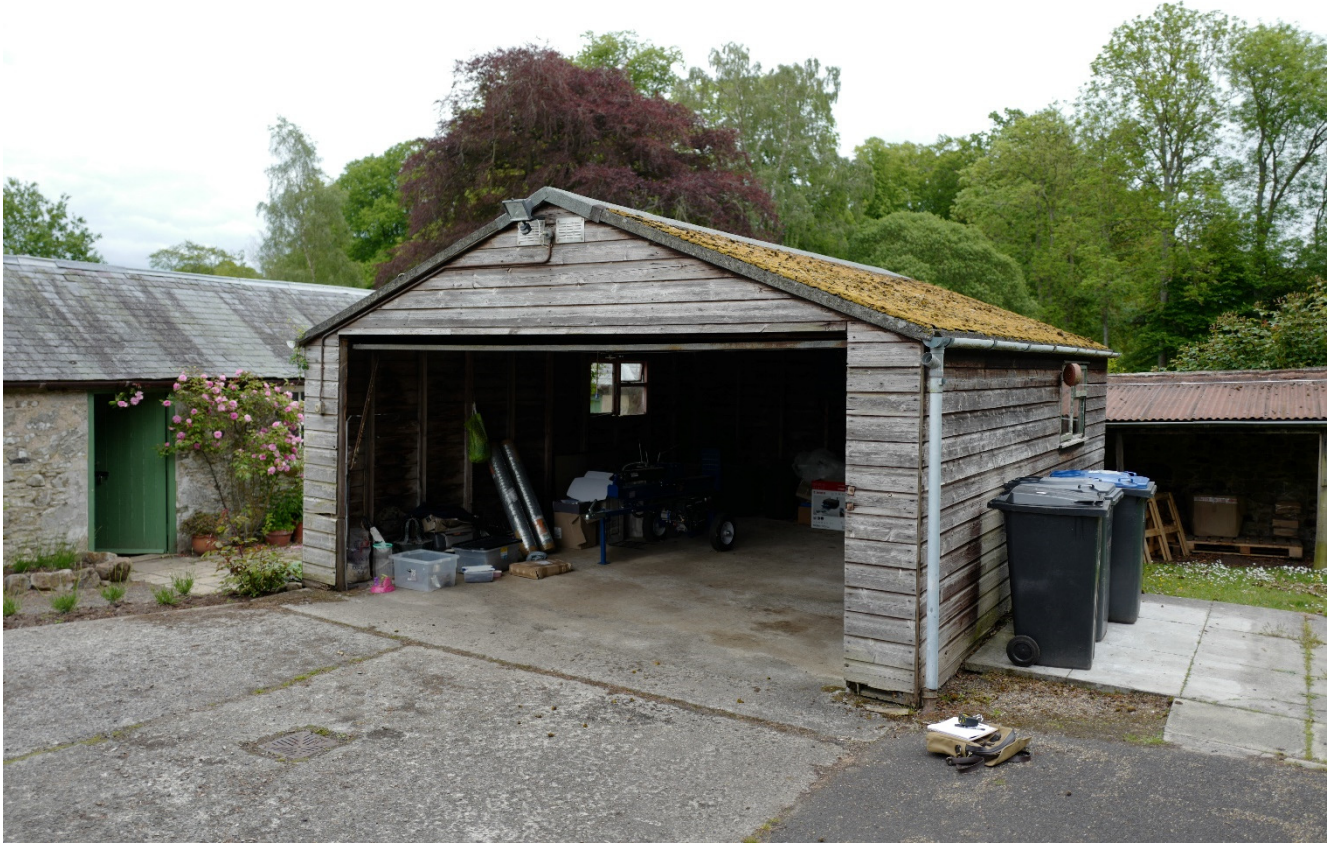
04 front elevation of existing garage
