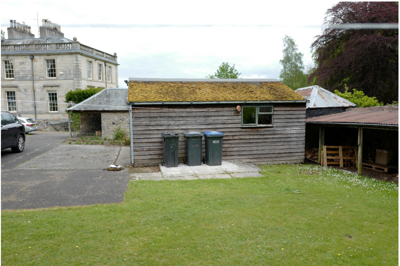
02 side elevation of existing garage with glenburn hall in background
