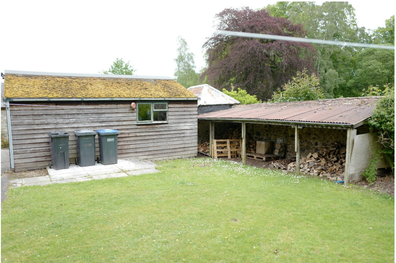
03 existing garage and log store
