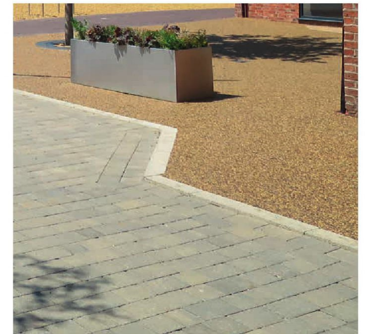
An example of carriageway/shared surface in resin bound gravel and block paving
