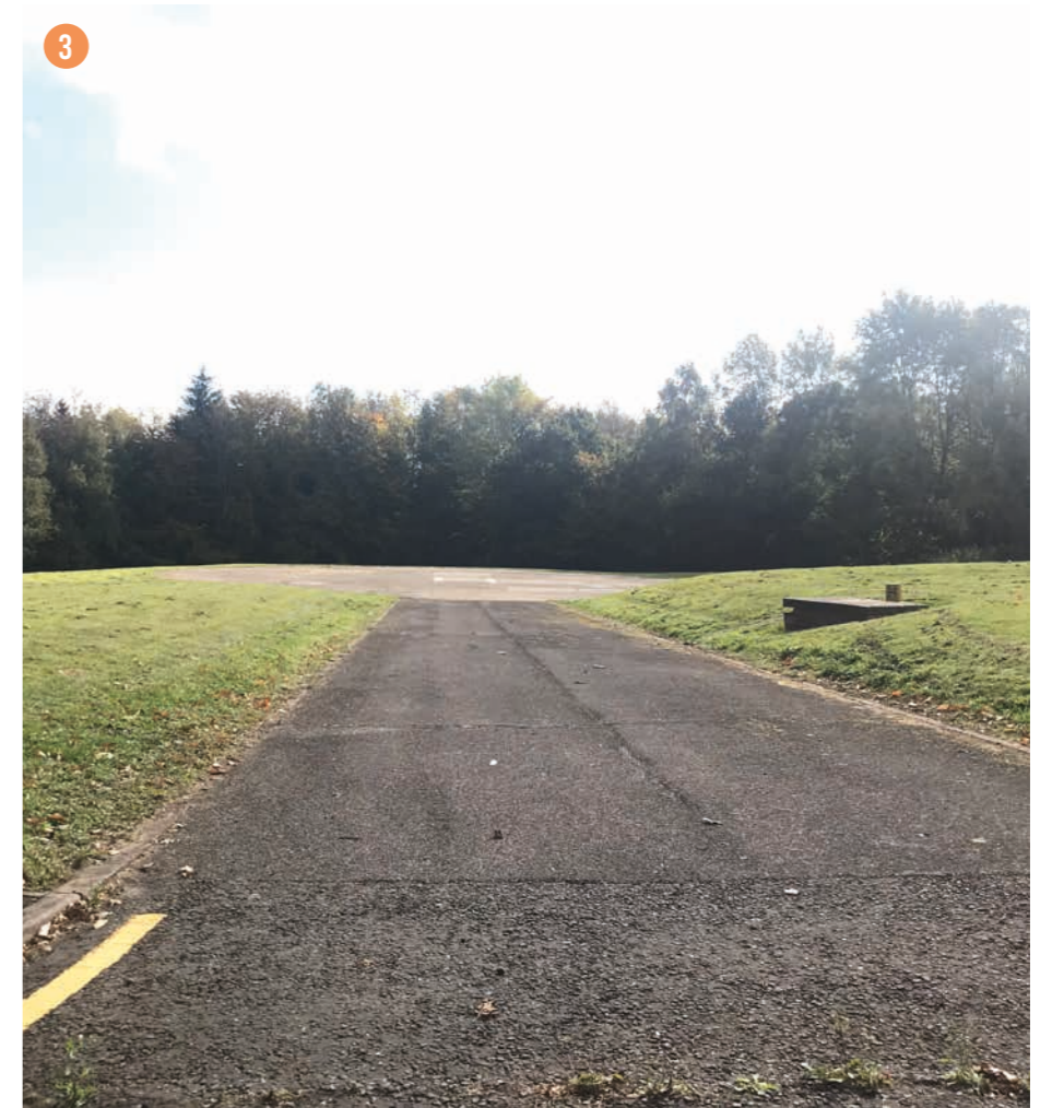
The helipad site
