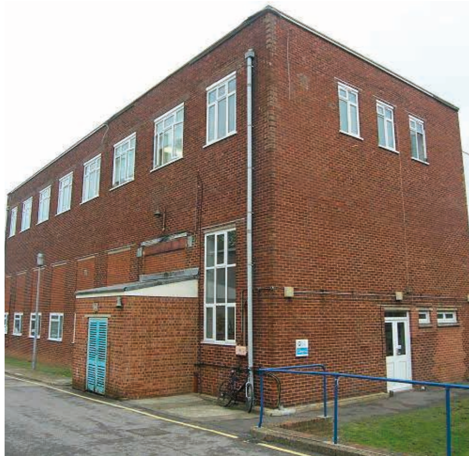
Building Q14/Penney Building (Grade II Listed Building)
