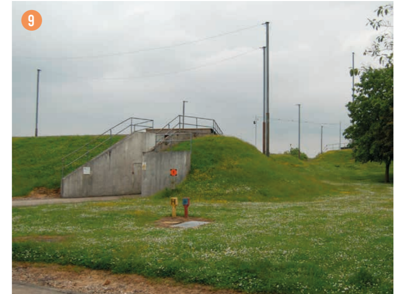
View of bunkers to be retained
