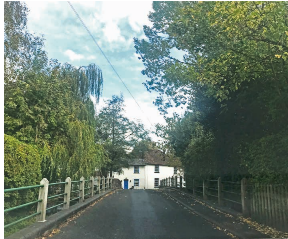
Bridge over River Darent
