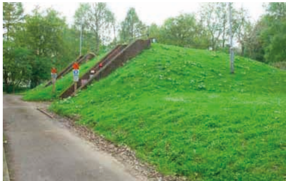
View of a bunker within the Fort
