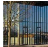
Large areas of glazing
