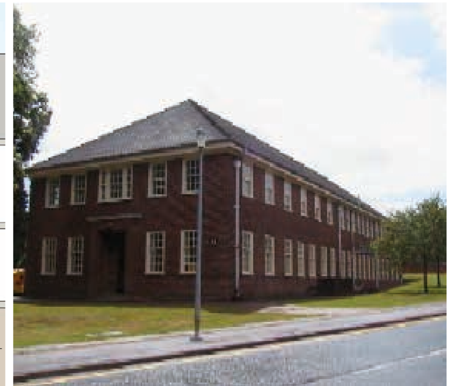
A1 building to be retained
