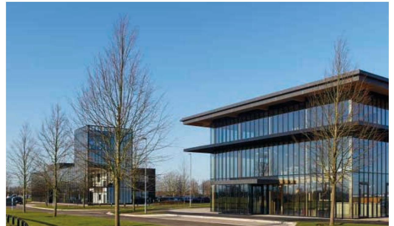
Office/R&D buildings at Alconbury Weald, Huntingdon
