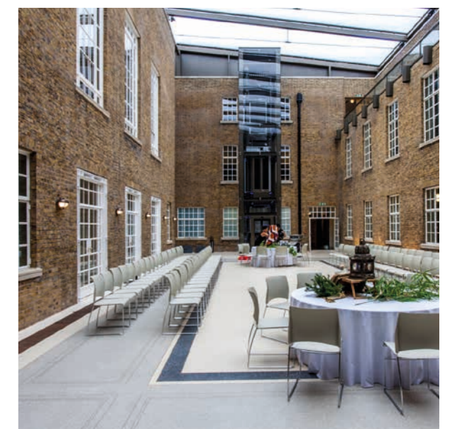
Glass lift abutting existing building (Hackney Town Hall)
