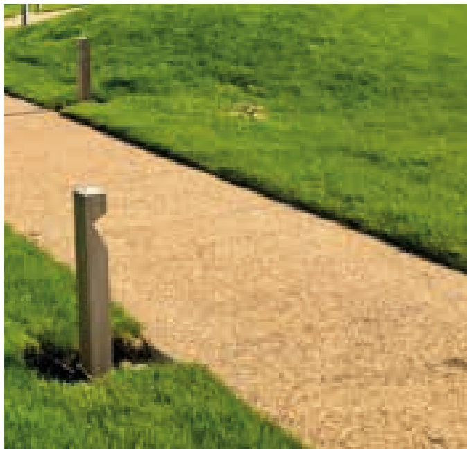
An example of formal open space footway/cycleway – buff resin bound gravel with aluminium edge restraint
