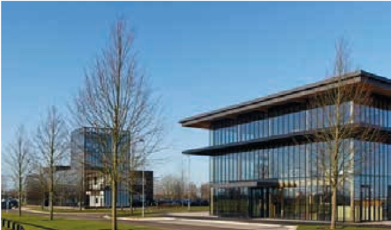
Office/R&D buildings at Alconbury Weald, Huntingdon
