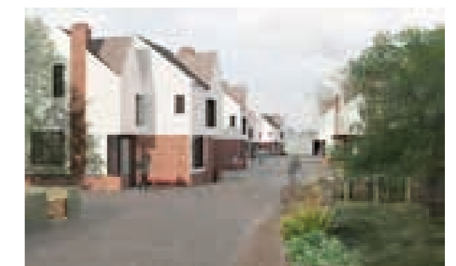
Precedent of lighter materials used to reflect more light (Lavenham, Housing by Project Orange).
