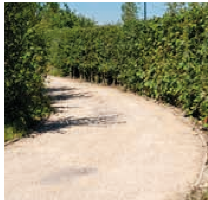
An example of informal open space footway – buff self binding gravel with timber edging
