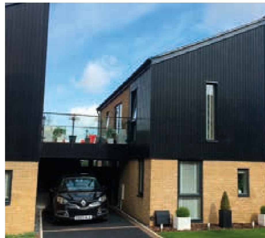
Precedent image showing a narrow fronted house type with first floor terrace (Newhall, Essex)
