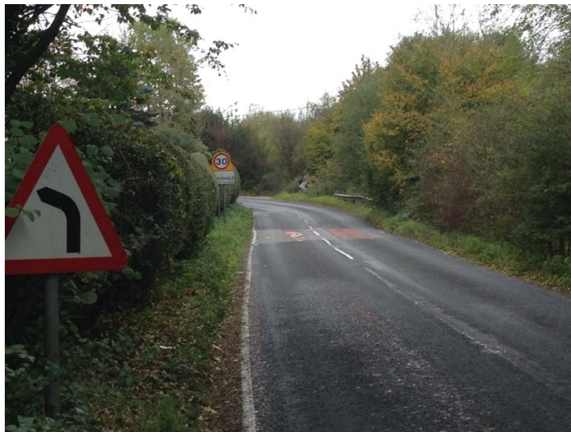
Photo 4: Faded entry treatment on entry to Knockholt Pound (south of Birchwood Lane)
