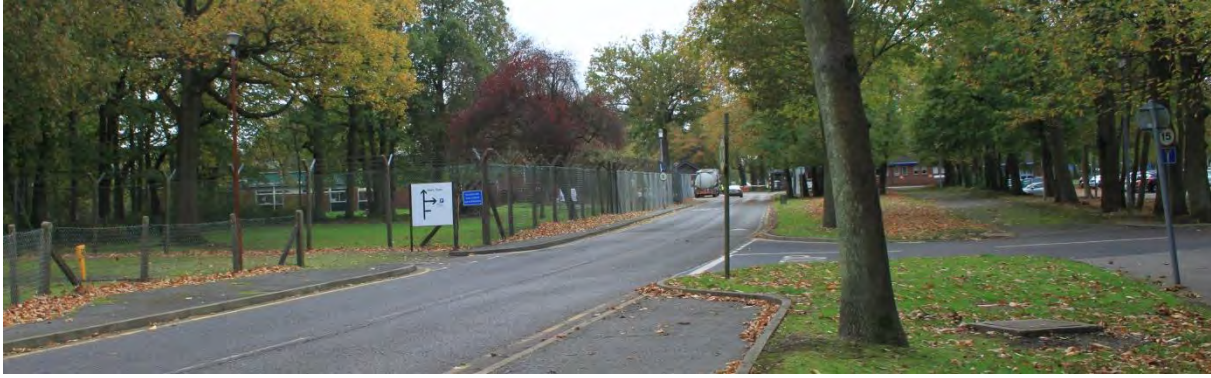
Figure 4.1 Fort Halstead Main Entrance Road, Crow Drive (Viewpoint 1)
