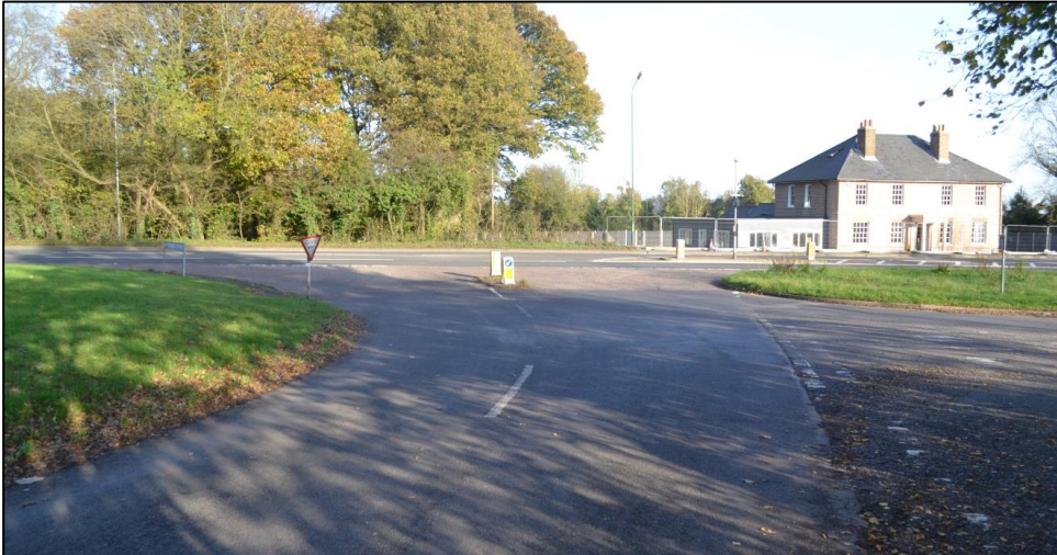
Figure 2-4 Main Access onto A224 Polhill from Otford Lane
