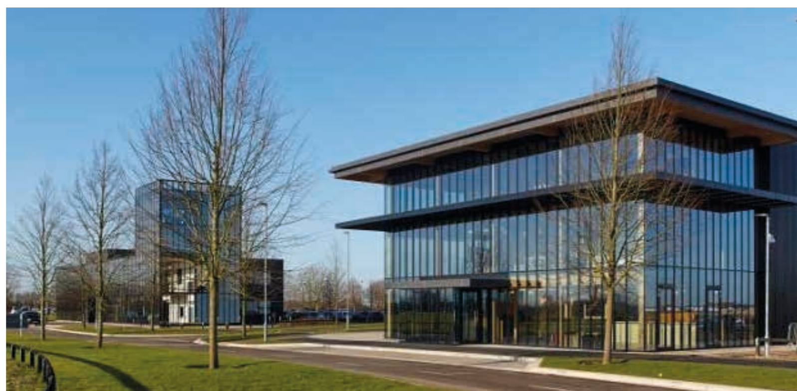
Office/R&D buildings at Alconbury Weald, Huntingdon
