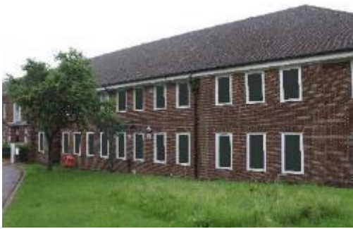
Plate 4.1: Brick building with hipped, tiled roof
