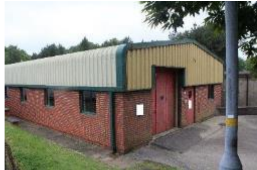
Plate 4.4: Brick building with pitched, corrugated metal roof and corrugated metal cladding
