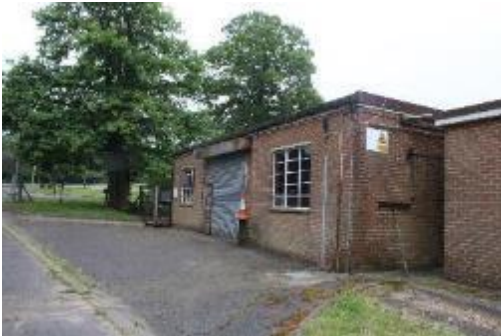
Plate 4.3: Brick building with flat, felt roof
