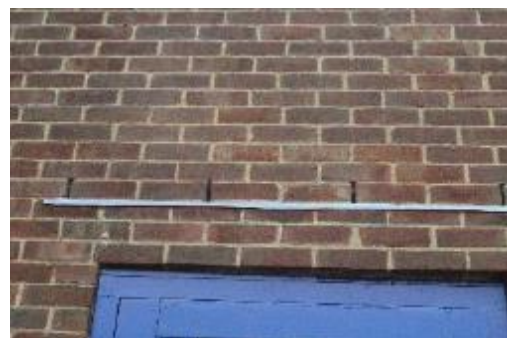
Plate 4.8: Weep holes in brickwork
