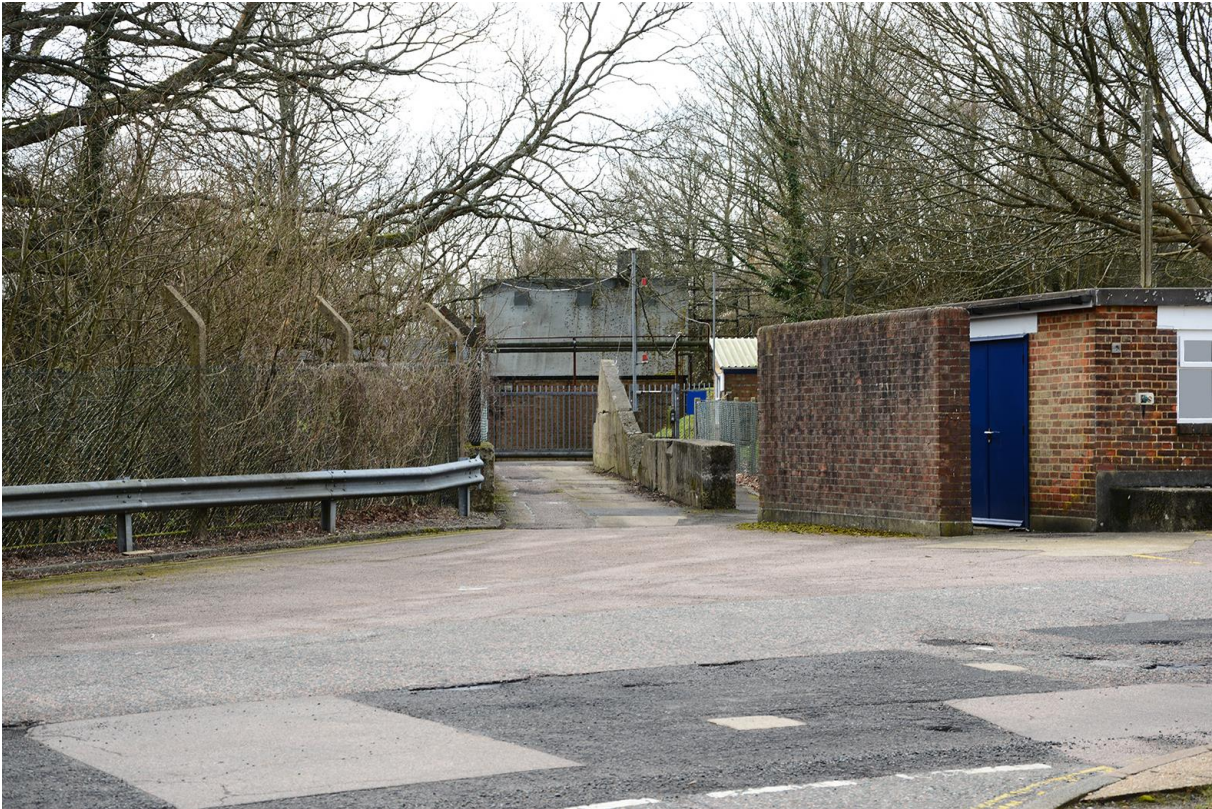
Plate 8: View looking towards the Fort's entrance
