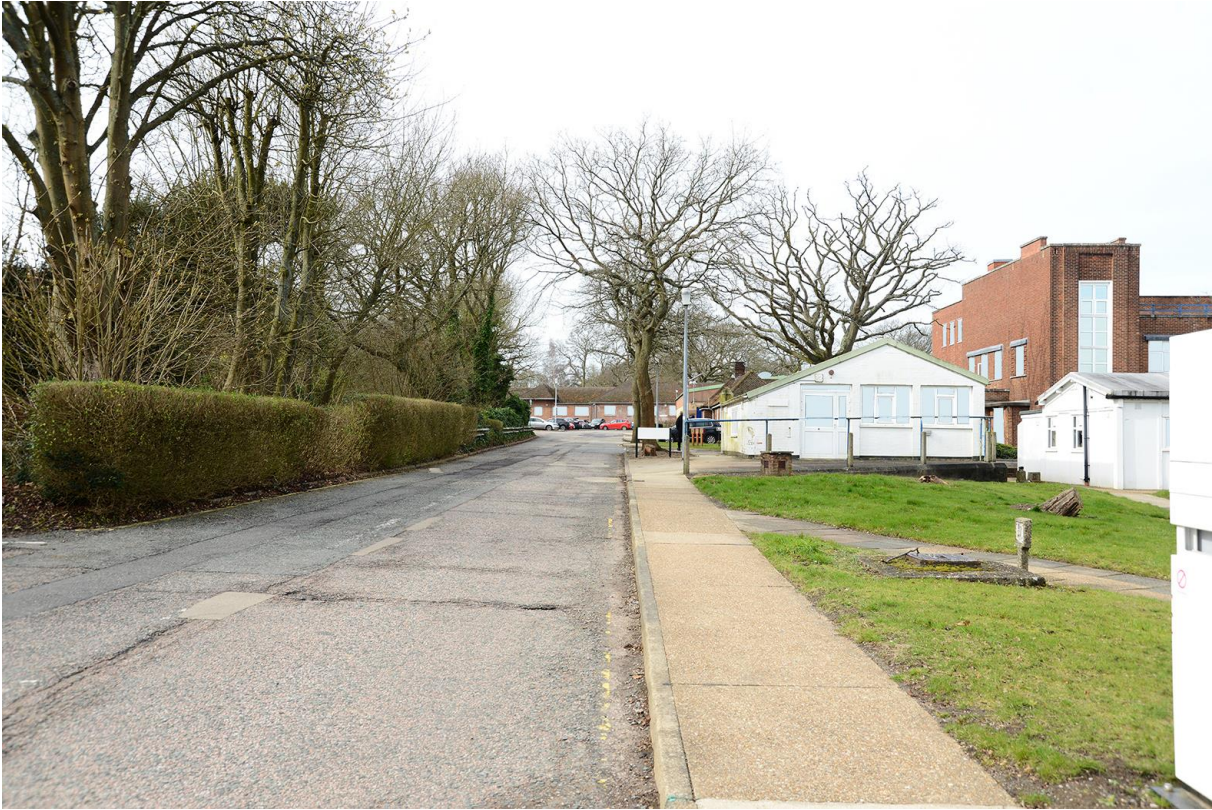
Plate 6: View looking east along Crow Road with the Fort on the left-hand side and the brick Q13 and Q14 visible to the right-hand side.
