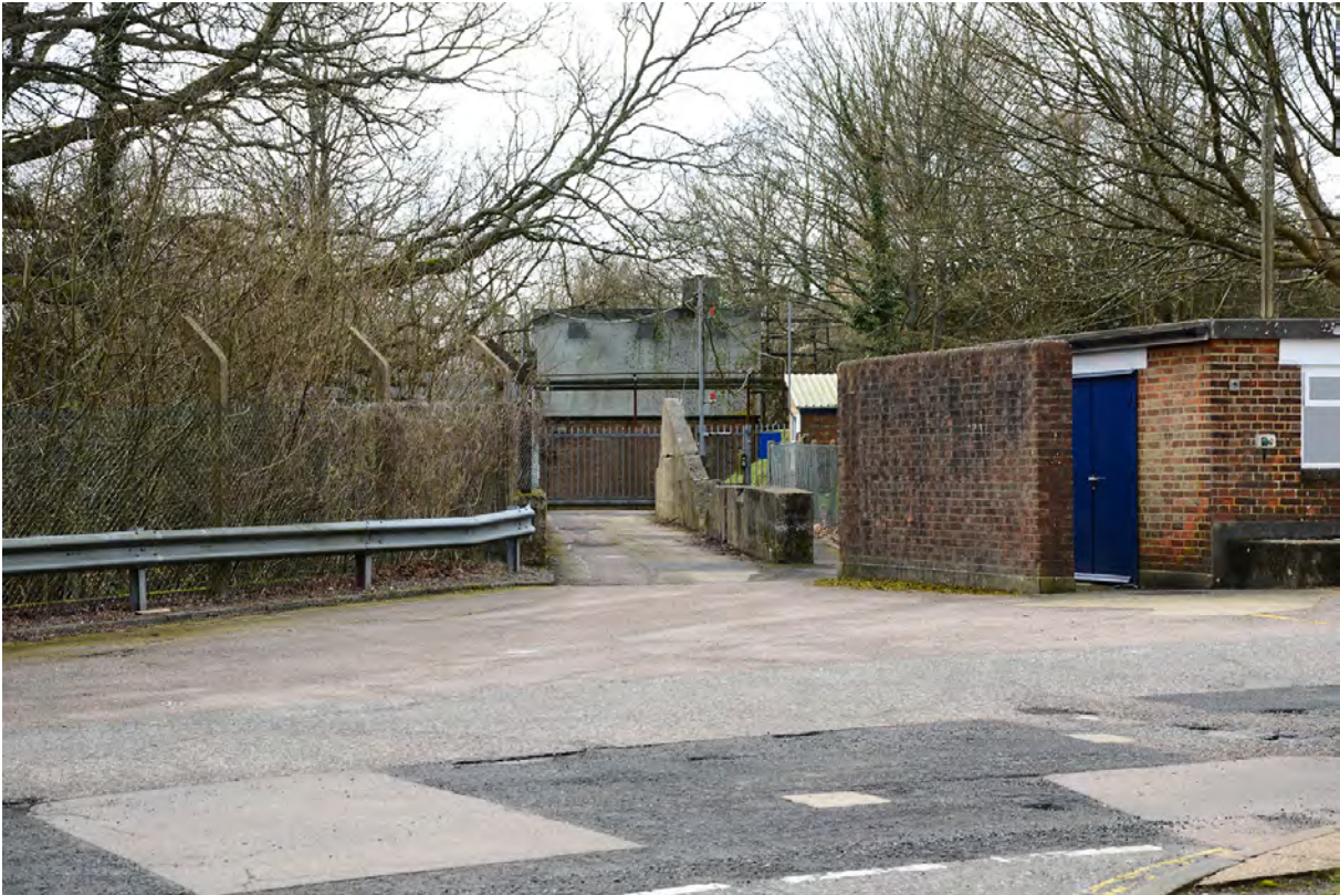
Plate 8: View looking towards the Fort's entrance
