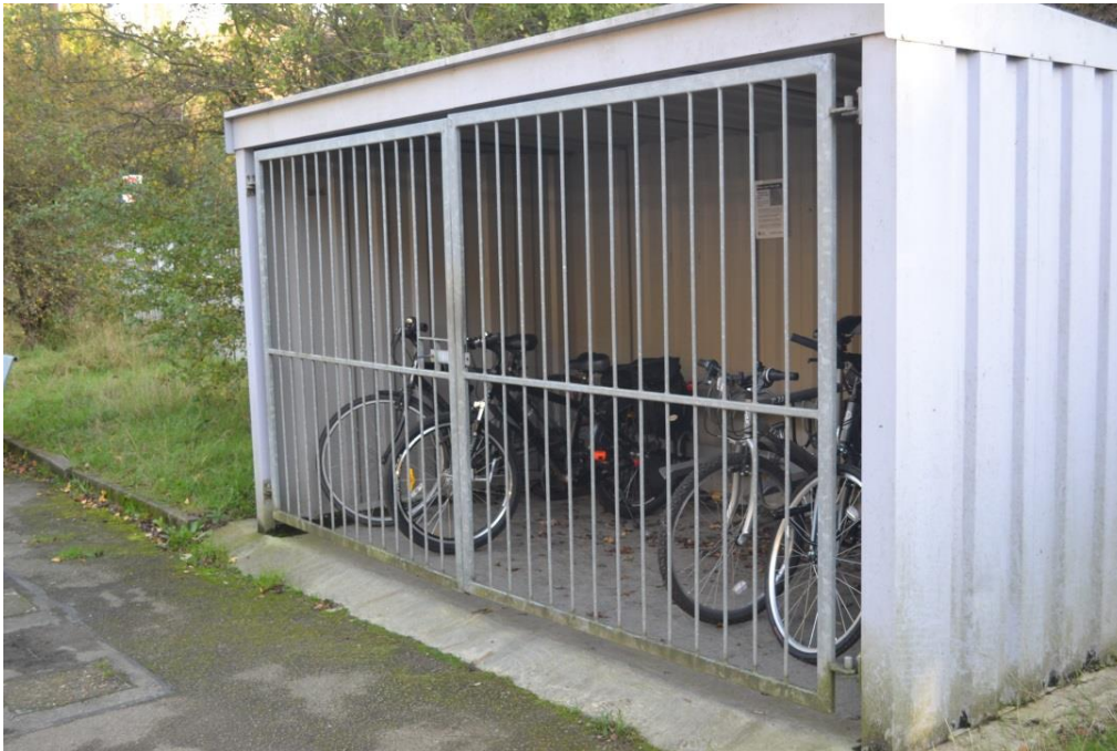
Figure 2-8: Cycle Parking at Knockholt Station
