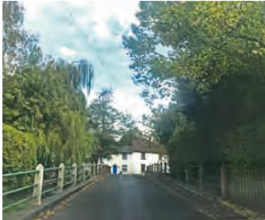
Bridge over River Darent
