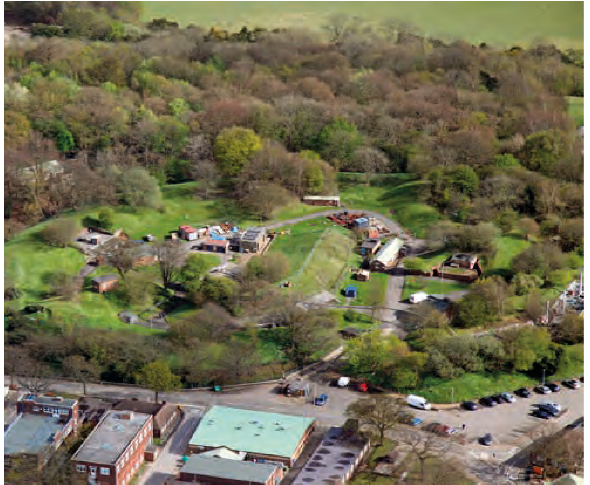
Aerial photograph looking South to the Fort
