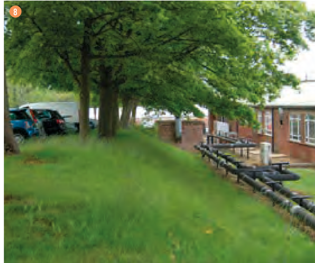
View of the ground level change along Crow Drive
