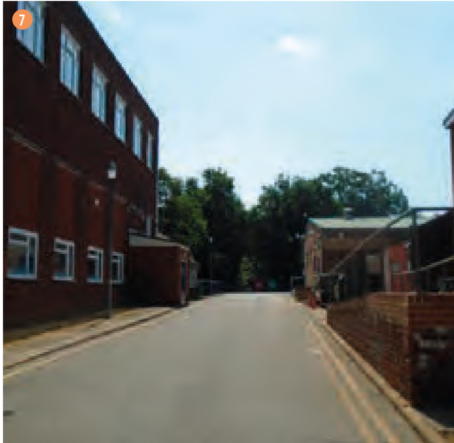
View of the ground level change next to Q14 Penney building
