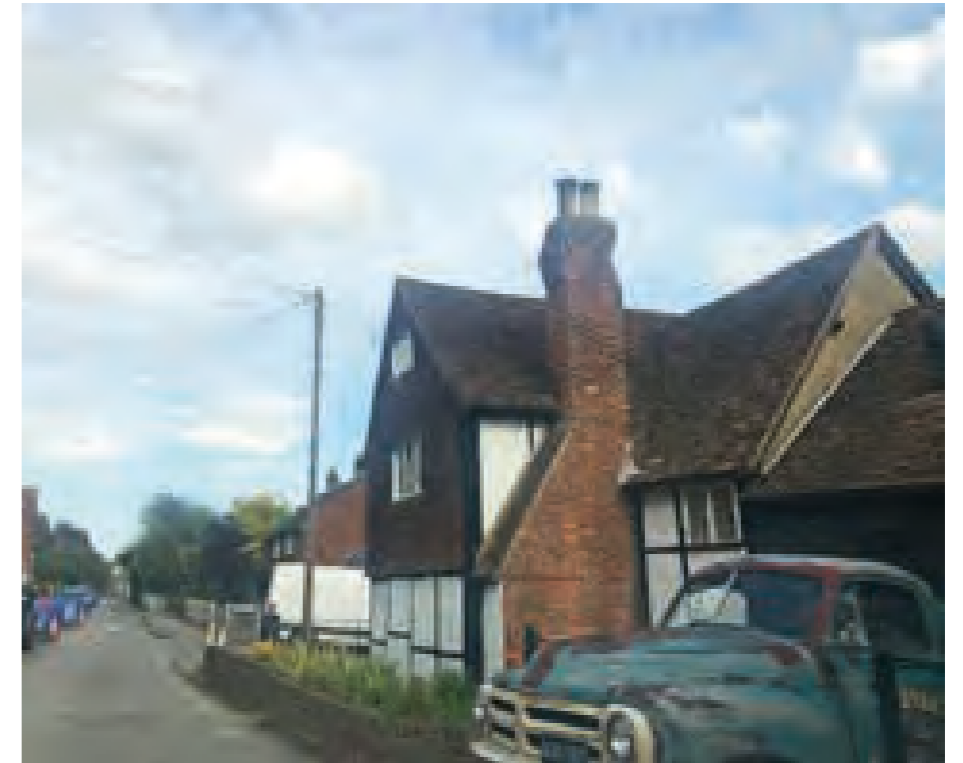
High Street 15 th century detached house, Grade II listed
