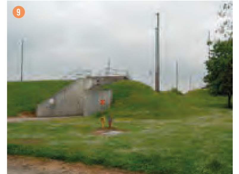
View of bunkers to be retained
