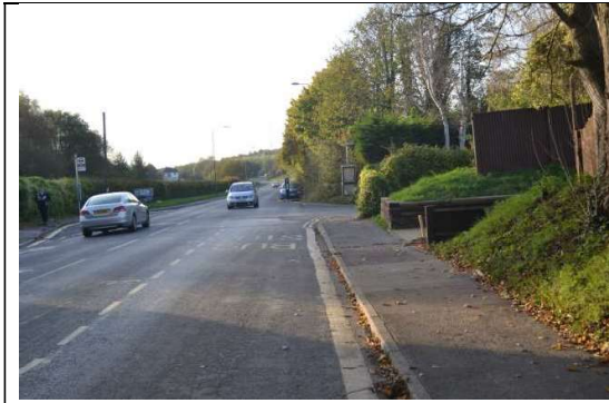
Photo 3: Old London Road at station access road
